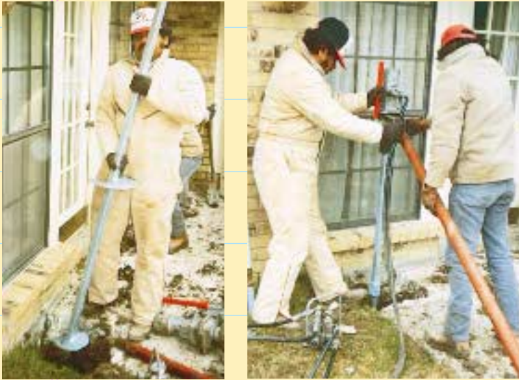
Chance's system relies on helical piers (left) inserted into holes around the foundation. Power equipment screws the piers into the ground (right) until resistance indicates that good bearing is achieved.
