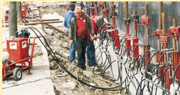
Ram Jack employs a sophisticated hydraulic lifting system for smoothly raising large, heavy structures.
