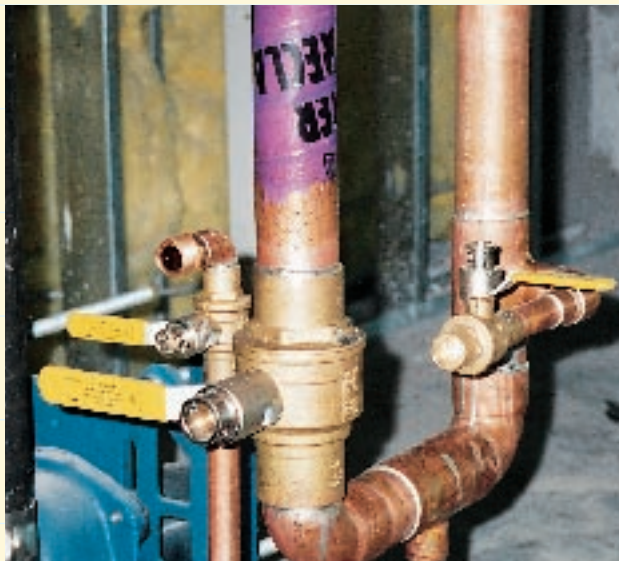
Purple tape on water piping indicates reclaimed, non-potable water.
