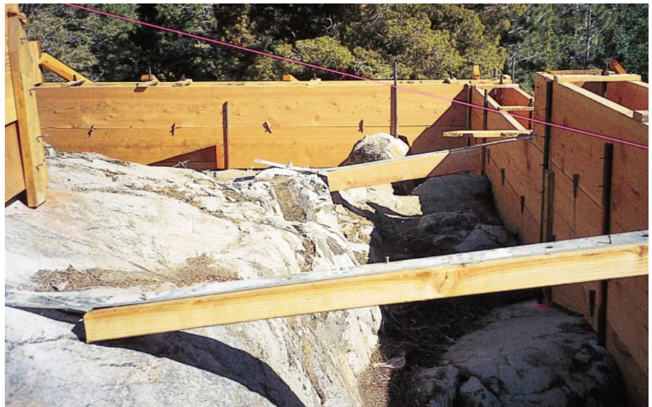
Figure 4. Simpson MST framing straps and 2x4 strongbacks, anchored with expansion bolts, braced the forms to the irregular rock outcroppings.
