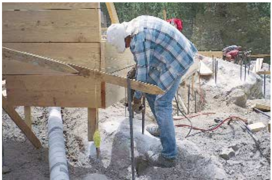
Figure 6. To protect against puncture and cracking, all utility lines were wrapped with a closed-cell foam wrapping (at left in photo).
