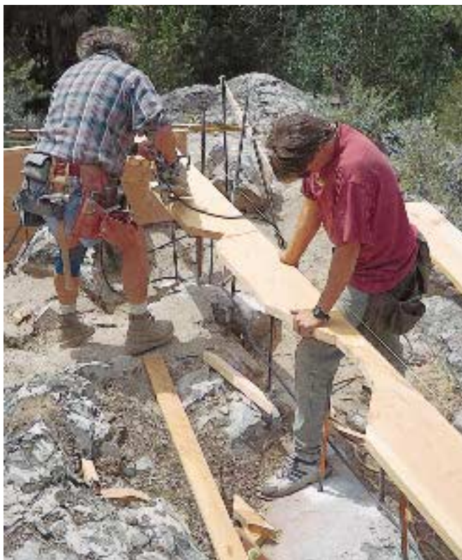
Figure 1. When working on ledge, even the batter board stakes must be supported in drilled holes.
