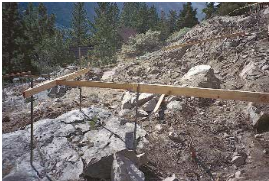
Figure 1. When working on ledge, even the batter board stakes must be supported in drilled holes.
