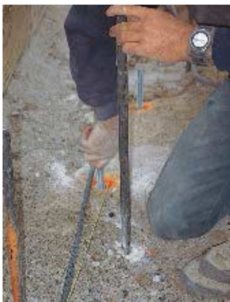
Figure 3. The author's crew used a Bosch rotary hammer to drill over 300 holes in the rock outcroppings (top left). After blowing the dust out of a hole (top right), they injected epoxy (bottom left). To ensure good coverage, they also coated the rod and worked it up and down in the hole (bottom right).
