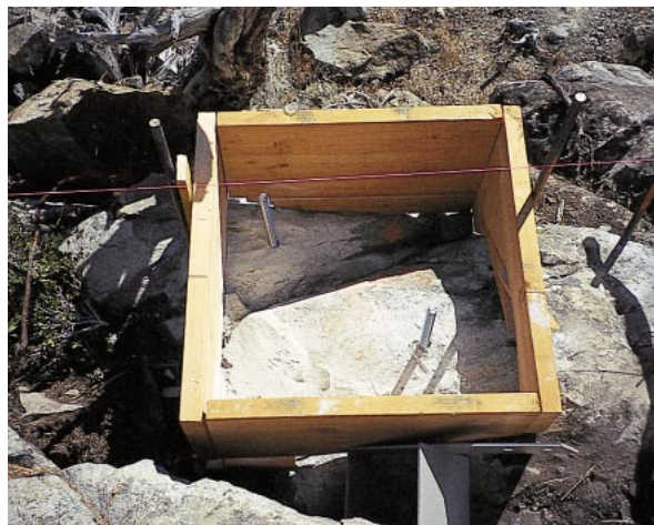
Figure 5. For pier footings, a flat surface was jackhammered into the ledge and two epoxied dowels inserted.
