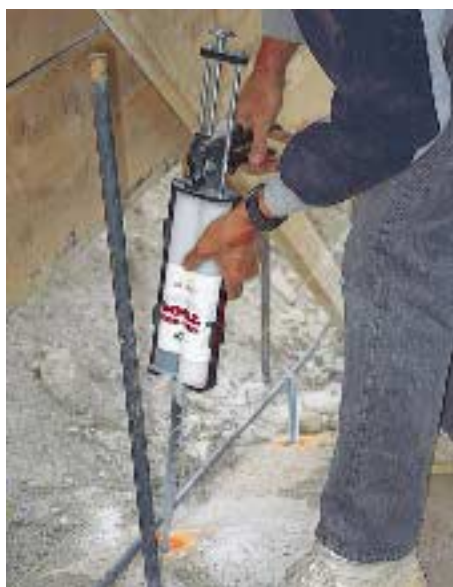
Figure 3. The author's crew used a Bosch rotary hammer to drill over 300 holes in the rock outcroppings (top left). After blowing the dust out of a hole (top right), they injected epoxy (bottom left). To ensure good coverage, they also coated the rod and worked it up and down in the hole (bottom right).
