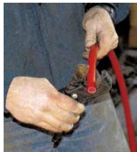
Figure 2. PEX tubing can be cut with a special scissorslike tool (above), or simply with a sharp pocketknife. A crisp, square cut is critical for a lasting joint.
