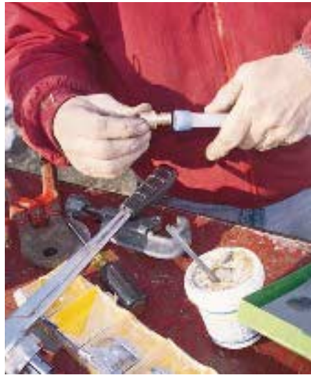
Figure 3. To make a simple joint using Wirsbo's method, you slide a PEX ring over the tube, expand the tube with Wirsbo's expanding tool (left), and quickly insert the fitting (right) before the PEX returns to its original diameter.
