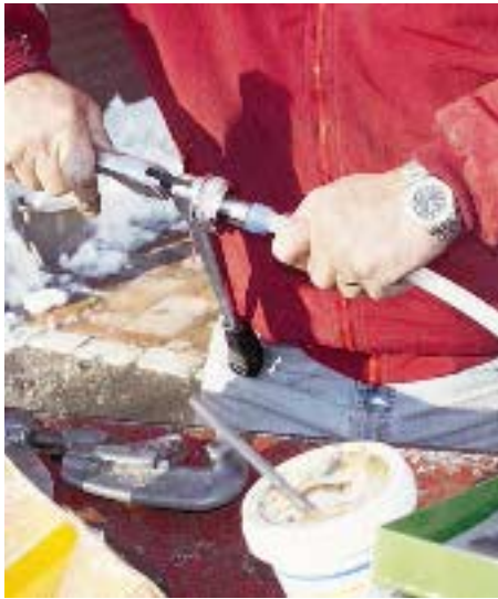
Figure 3. To make a simple joint using Wirsbo's method, you slide a PEX ring over the tube, expand the tube with Wirsbo's expanding tool (left), and quickly insert the fitting (right) before the PEX returns to its original diameter.
