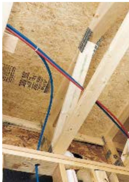
Figure 6. Various clips and supports are available from pipe manufacturers to help support PEX runs (above). Where possible, individual tubes should be bundled together for support and a neat appearance (left).
