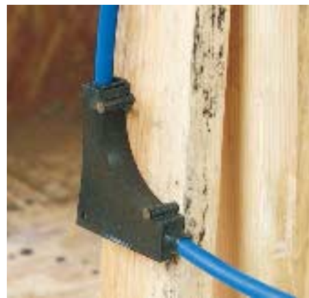
Figure 6. Various clips and supports are available from pipe manufacturers to help support PEX runs (above). Where possible, individual tubes should be bundled together for support and a neat appearance (left).
