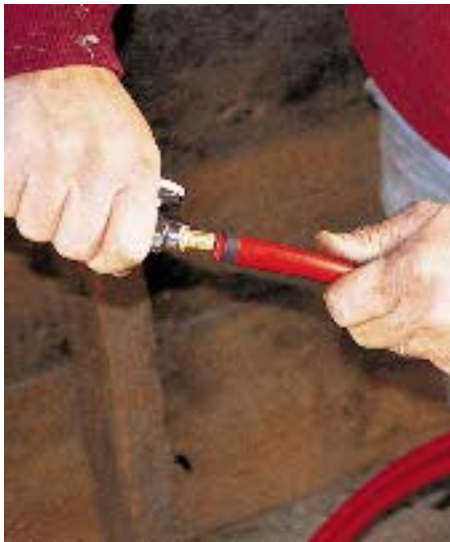
Figure 4. In the Vanguard joint system, tubing slides over the fitting without expanding (left) and is secured with a copper crimp ring. Crimping with Vanguard's crimping tool takes only a few seconds (right).
