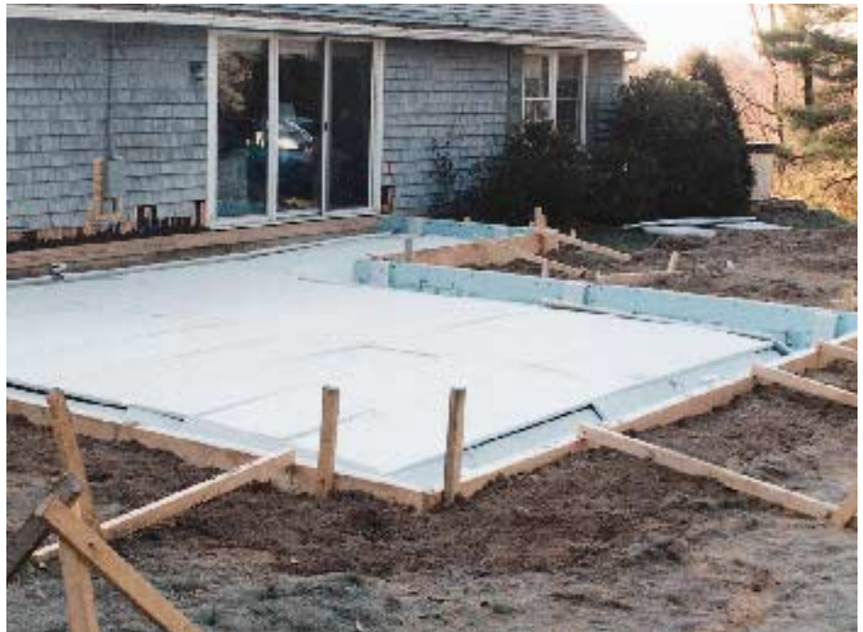
Ready to pour. After the sand base is compacted, 1-inch-thick foam board is laid over the entire subgrade and in the footing trenches. The forms have been backfilled to prevent movement during the pour. Note the pressure-treated 2x6 screed attached to the house.
