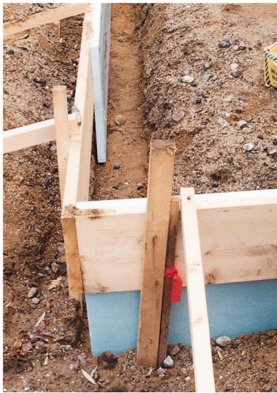
Insulated formwork. Two-by-twelve form boards are lined with 1½-inch-thick extruded polystyrene insulation board. The author digs the footing trench a full 24 inches deep (inset) to make use of the full width of the foam board insulation.
