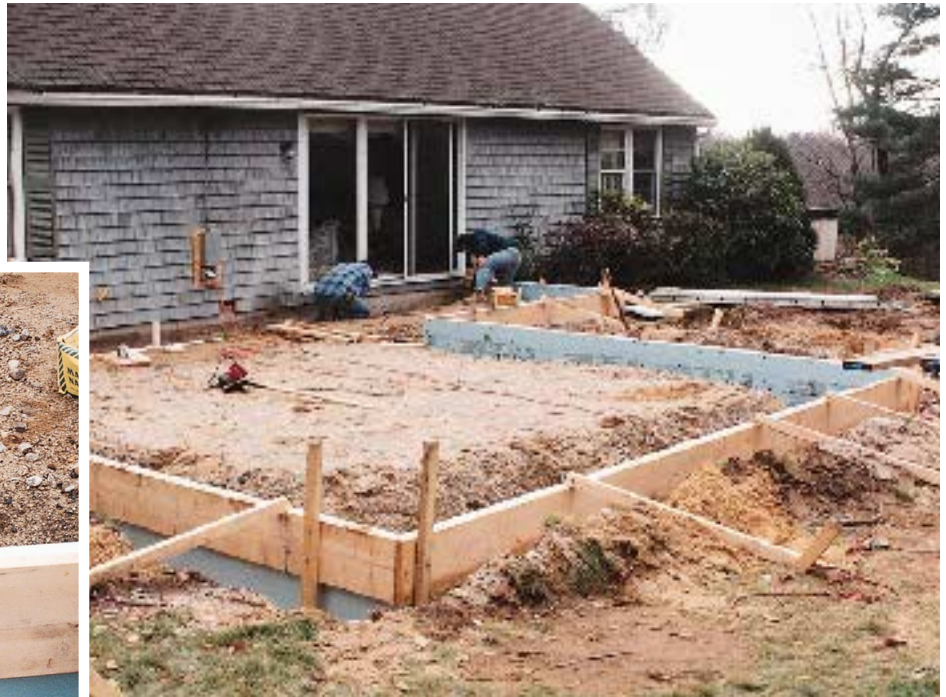
Insulated formwork. Two-by-twelve form boards are lined with 1½-inch-thick extruded polystyrene insulation board. The author digs the footing trench a full 24 inches deep (inset) to make use of the full width of the foam board insulation.
