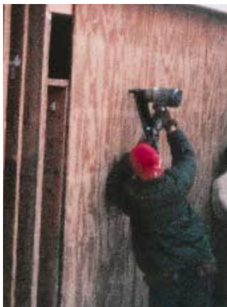
Figure 4. Joist hangers were used at the top of studs to resist the thrust of the fill (above). The PT plywood was run vertically, to avoid the need for blocking (left).
