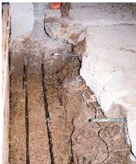
Figure 2. In the new footings, horizontal rebar was tied both to the basement foundation and to pins drilled into the existing slab.
