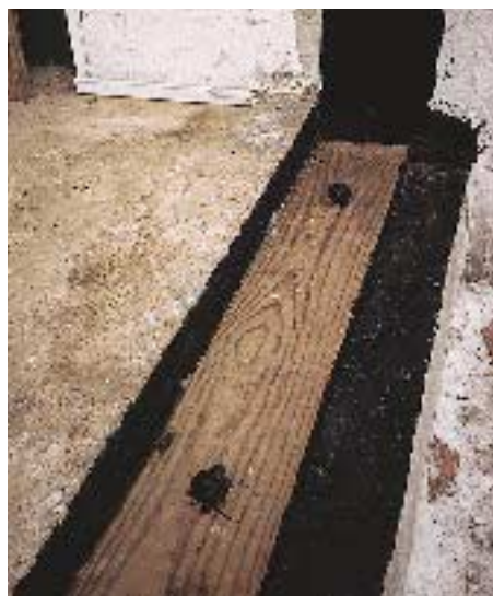
Figure 3. A trowel-applied foundation coating keeps the PT sill from wicking moisture from the footing.
