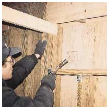
Figure 4. Joist hangers were used at the top of studs to resist the thrust of the fill (above). The PT plywood was run vertically, to avoid the need for blocking (left).
