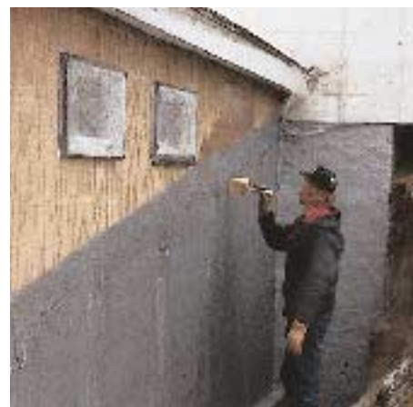
Figure 5. To prevent leaks, the author coated below-grade PT plywood with a rubberized coating, then sprayed it with a clear UV-resistant finish.
