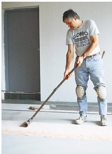
Figure 1. A tilesetter uses a floor roller to adhere a crack isolation membrane over a slab control joint. The membrane should be three times the width of the tile.
