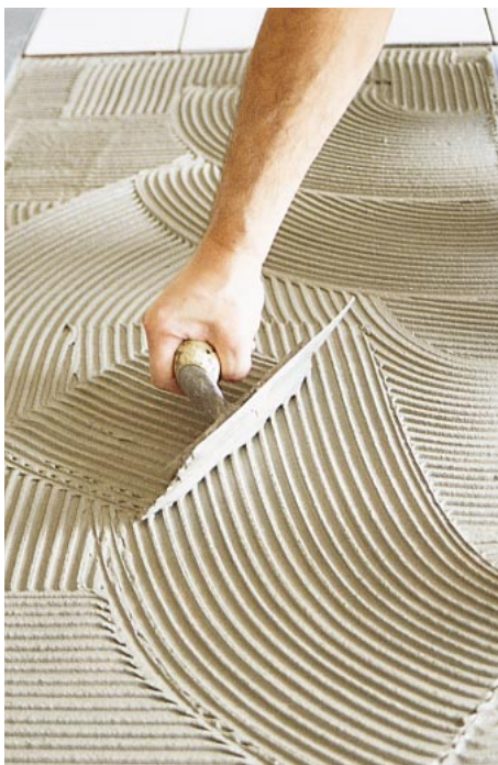
Figure 5. After applying the setting adhesive with the straight edge and bottom of the trowel, the tilesetter combs the setting bed with the trowel held at a 45-degree angle.
