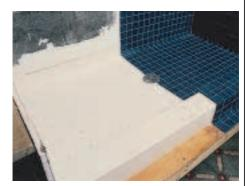
the plastic pan and can be set as soon as the module is in place. The back and sides are 6 inches tall and have a  $^{1/2}$ -inch lip to receive cement board or drywall. There's a  $4^{1/2}$ -inch preformed curb on the front, and the bottom slopes to a molded drain. Modules come in a number of sizes and have a lifetime guarantee against leakage. A 37x37-inch unit costs \$270.
