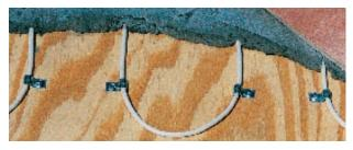
weight concrete. According to the manufacturer, Delta-Warm is suitable for use with any floor covering, including ceramic and vinyl tile, marble, concrete, carpet, and wood. Supplied in standard factory-terminated lengths, the installation cost runs between \$4 and \$16 per sq. ft., depending on the size of the area to be heated.
