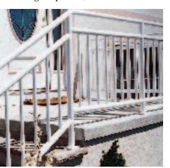
rise/run, stair radius, inside and outside corners, and other design considerations. All components are prefabricated and shipped preassembled; oversize systems are provided in smaller sections that are then fit together on site. The seamless railings are coated with a durable high-gloss finish to resist corrosion, even when exposed to salt air, and are mounted over steel brackets. All fasteners are concealed. Available in white (round stock also comes
