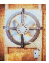
ly, according to the manufacturer. Instead of encasing the fan blade in a solid cylinder, the gable-mounted Whisper Cool automatic power ventilator employs a series of rings that are said to allow air to flow with less restriction. The fan
