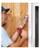
other half is getting it to cure properly. *Lifetime Universal Brand Caulk* has been reformulated so it will cure at temperatures between 0°F and 120°F. (Most water-based sealants will fail if the temperature dips below 40°F before they have time to cure.) The siliconized acrylic sealant will adhere to primed and unprimed wood,
