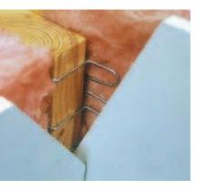
To avoid these problems, check out R-Plus Warm Corner Framing Clips. These galvanized steel clips, attached to corner studs or top plates at 16 inches on-center, create a backing for drywall panels. They're installed by hand, and don't need any fasteners, since the second corner panel wedges the first panel against the clips. In fact, corners constructed this
