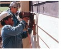
Smart Lap is a new composite lap siding made of specially shaped wood chips that are chemically united with a polyurethane binder. This engineered board is reportedly more dimensionally stable than a piece of solid wood siding. Smart Lap is also impreg-
