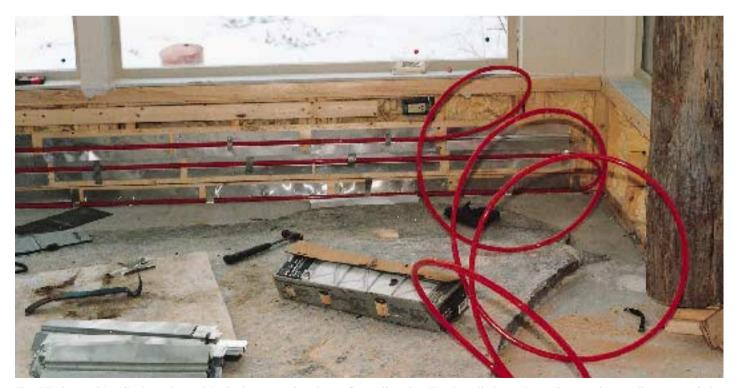
The PEX heat tubing fits in a channel in the heat transfer plates. On wall and ceiling installations, the author staples small squares of aluminum flashing over the tubing to hold it in place.
