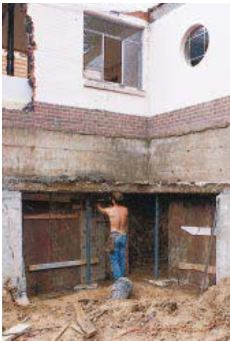
In this remodel, the foundation of the existing ranch was shored and a full basement added under the adjacent garage addition.
