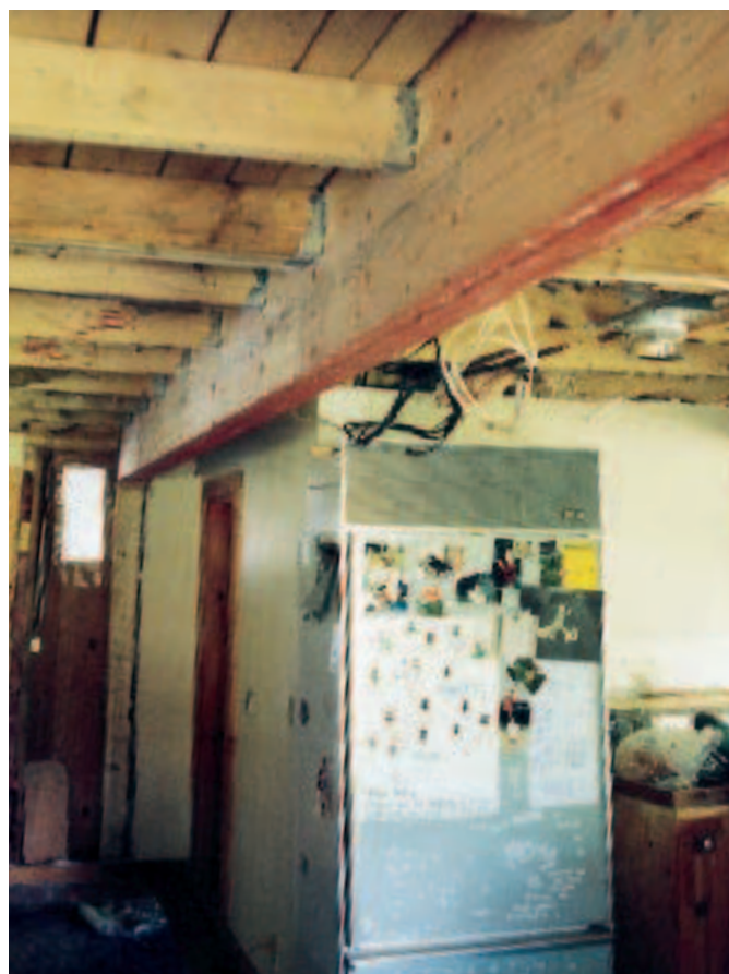
Figure 3. The LVLs were cut to length outside, slid through an access hole cut in the exterior wall, and nailed together in place. The steel hangers used to fasten the existing joists to the new beams made for a sleek appearance when the beams were wrapped in drywall.
