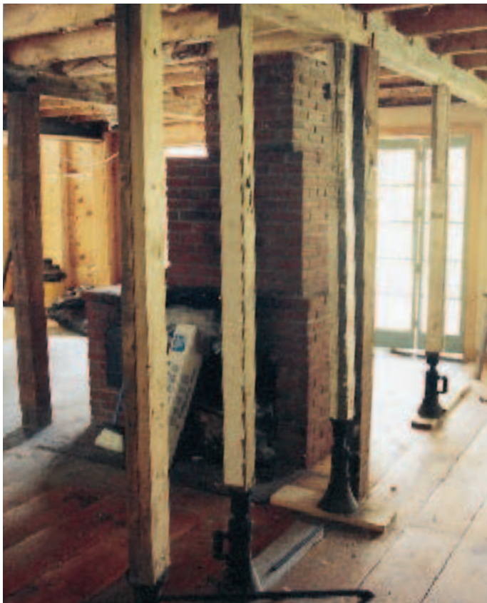
Figure 2. The old beams were first jacked to within \frac{3}{8} inch of level (left), then a temporary 2x4 bearing wall was built on either side, with each stud aligned directly under a second-floor joist (right). To maximize headroom, a section of each existing joist was cut out to make room for an inset 5\frac{1}{4} -inch-wide by 14-inch-deep LVL beam.
