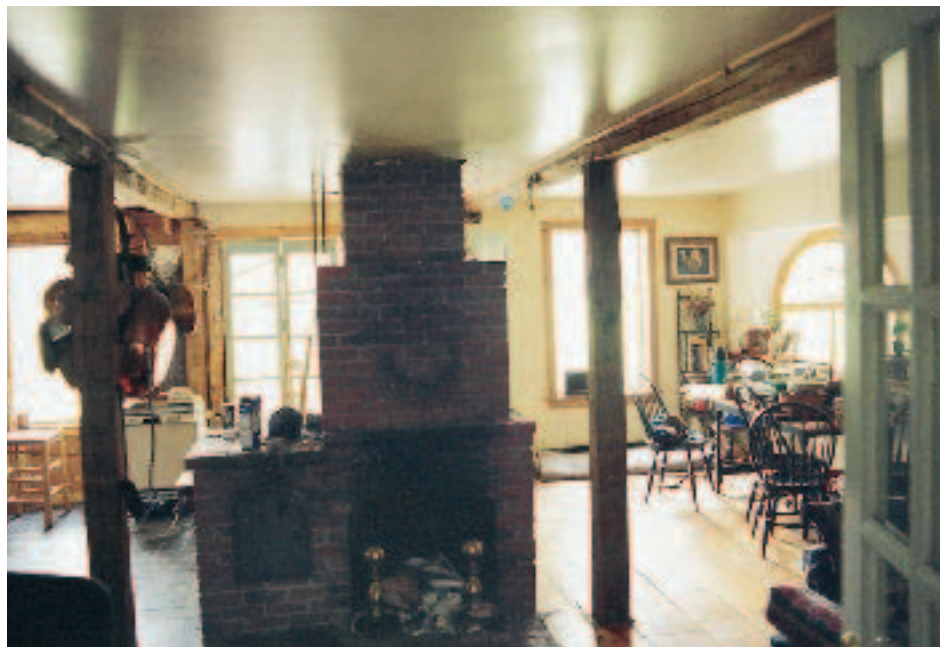
Figure 1. The 8x8 carrying beams were spliced over posts that interfered with the design for a kitchen addition and dining room renovation. To avoid the demolition and rigging required to replace the sagging 8x8s with steel, the author opted for built-up replacement beams made of LVLs fastened together in place.
