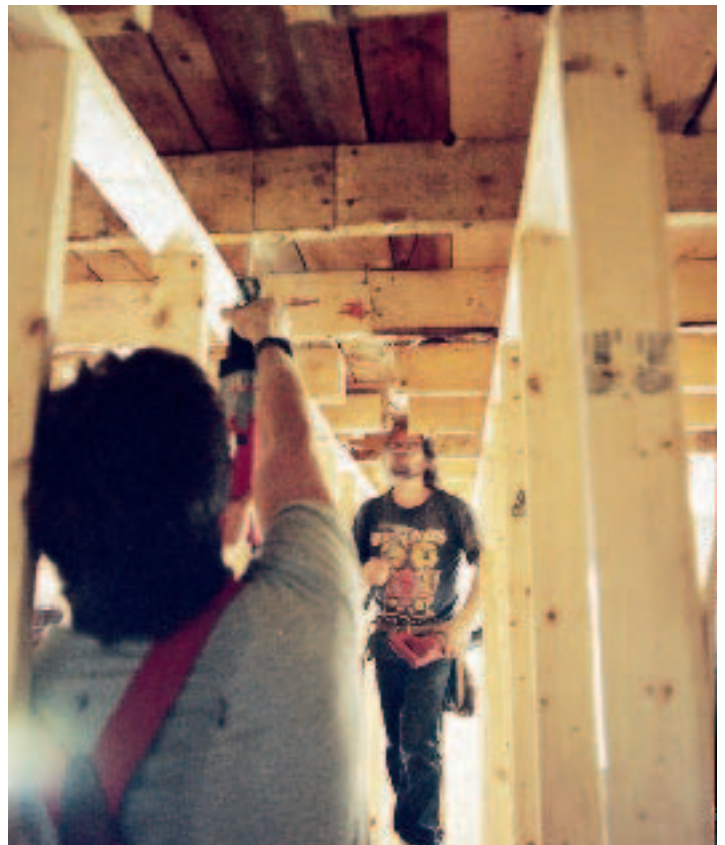
Figure 2. The old beams were first jacked to within \frac{3}{8} inch of level (left), then a temporary 2x4 bearing wall was built on either side, with each stud aligned directly under a second-floor joist (right). To maximize headroom, a section of each existing joist was cut out to make room for an inset 5\frac{1}{4} -inch-wide by 14-inch-deep LVL beam.
