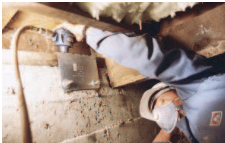
Figure 2. The Simpson FA series anchors are useful in tight quarters for anchoring the mudsill to the foundation wall. The side plate bolts to the foundation wall with epoxied threaded rod; the top can be nailed with a palm nailer.
