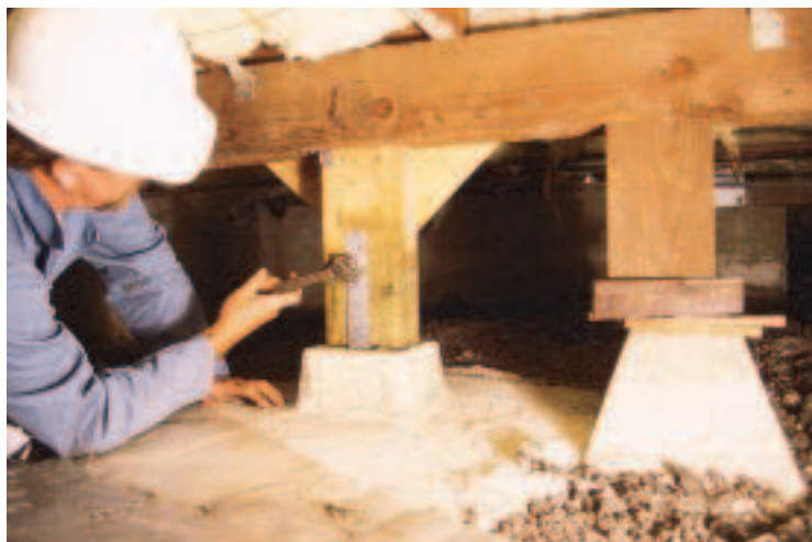
Figure 4. New post-and-pier supports are built in place using precast pier blocks set in a 2-foot-square concrete footing. Note how the original post, at right in the photo, has no mechanical anchorage.
