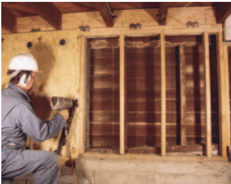
Figure 3. In cases where the old foundation is too weak to hold anchors, it's necessary to pour a new wall. In the case shown here, a new stepped stem wall was poured tight to the existing one, with new cripple walls built on top. Simpson A35F clips secure the cripple wall to solid blocking between the floor joists above (see photo).
