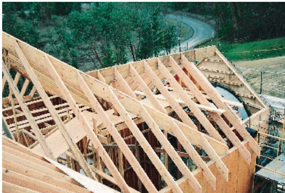
Figure 4. Because the main hip interrupts the gable rafters (above), the upper jacks will meet high on the hip (left) to stay in plane with the lower jacks.
