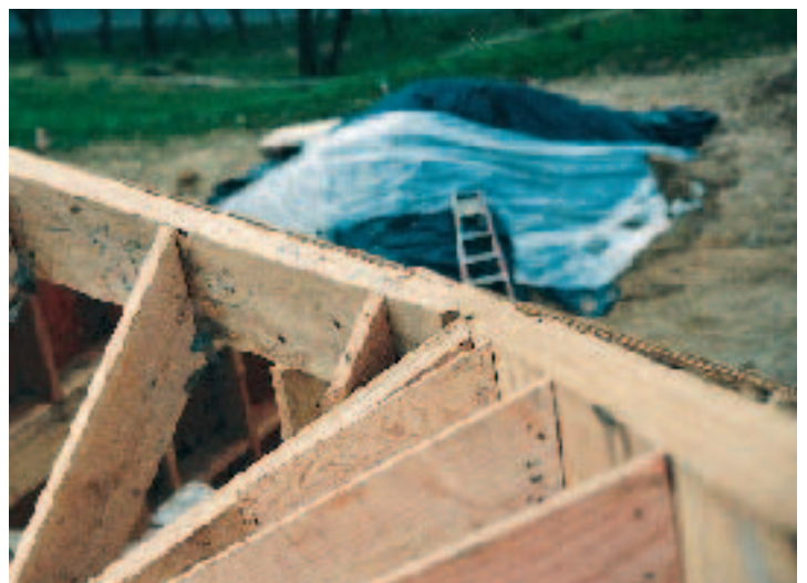
Figure 3. A special cheek cut is required to align the ridge with hip and valley beams of different thicknesses (photo). First, lay out a standard double 45-degree cheek cut, then add 7/8 inch (half the difference between the two beam widths) to the side towards the thinner material (illustration).
