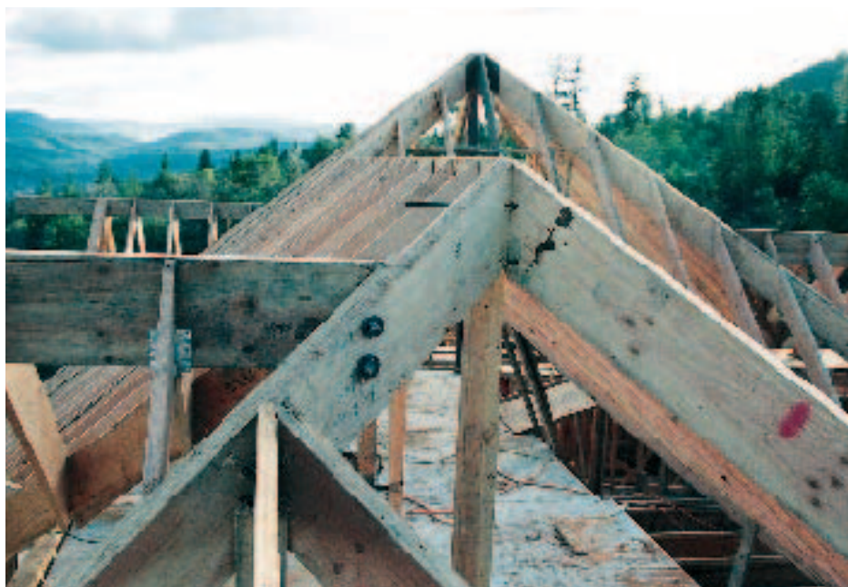
Figure 6. When a single beam serves as both a valley and a hip, it must be backed. The right side of this valley (valley #3 in Figure 1) is backed from the valley-to-valley connection up to the ridge, and on the left side from the ridge back down to the gable ridge (coming in from the left side in the photograph). These rips can be made on the ground or in the air after the roof has been stacked.
