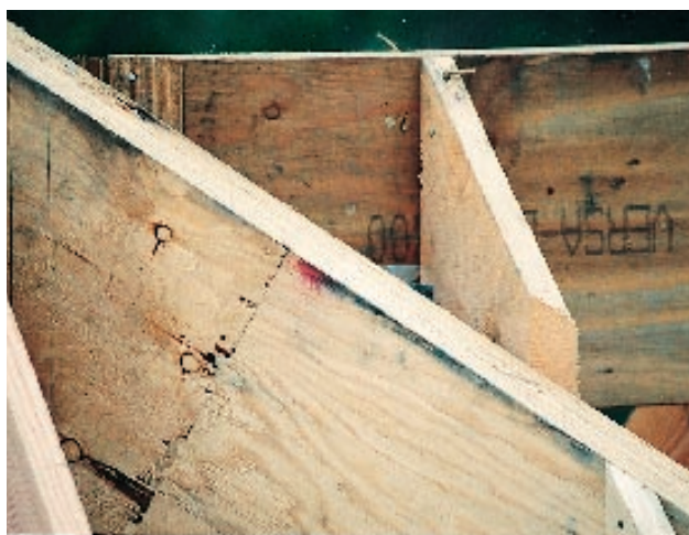
Figure 4. Because the main hip interrupts the gable rafters (above), the upper jacks will meet high on the hip (left) to stay in plane with the lower jacks.
