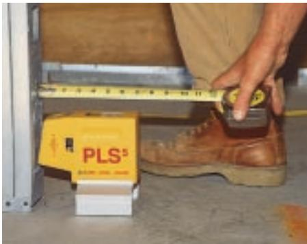
**The vertical beams of the PLS-5 laser can be used to establish plumb lines to the ceiling from layout marks on the floor. The beam is strong enough to be visible on a tape measure, making it easy to check in-place work for alignment.**
