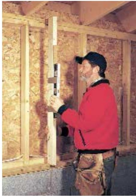
The author uses a custom-made level to make sure he's plumbing wall plates instead of individual studs. With proper calibration, even a crooked stick and a broken level will give accurate readings.
