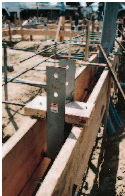
Figure 3. The author uses plywood templates (photo, above) or Simpson “Monkey Paws” (drawing) to secure hold-down bolts to foundation form boards. Embedded strap anchors are tacked into place, while post anchors (left) are temporarily secured to a scrap of framing lumber of the correct width.
