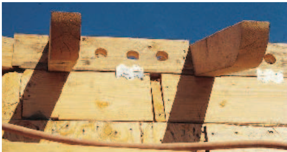
Figure 6. Here, Simpson A35F clips tie eaves blocking to the ceiling diaphragm below.
