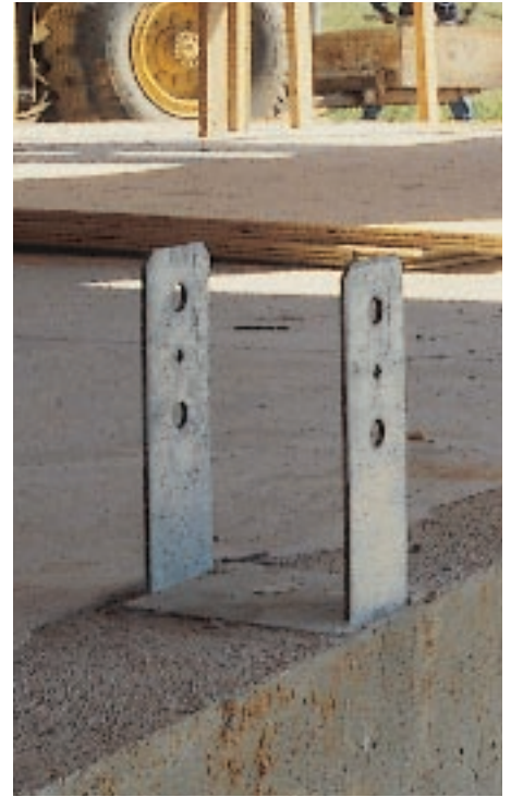
Figure 2. Bolts for hold-downs like the type in the photo above, left, have to be precisely located with respect to the framing when the foundation is poured, as do post anchors (above). Embedded straps (left) are somewhat more forgiving.
