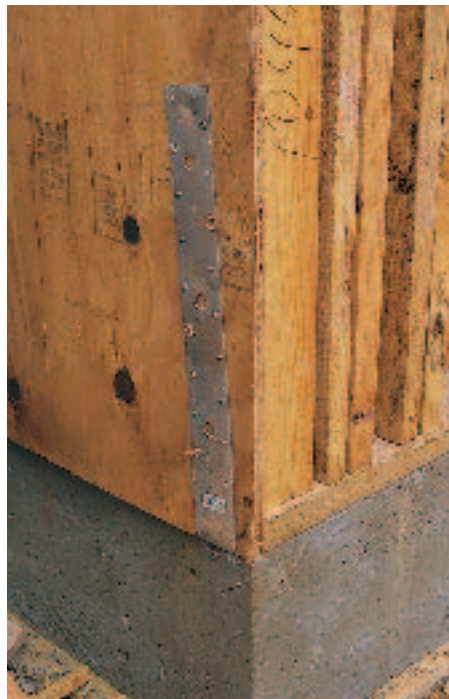
Figure 2. Bolts for hold-downs like the type in the photo above, left, have to be precisely located with respect to the framing when the foundation is poured, as do post anchors (above). Embedded straps (left) are somewhat more forgiving.
