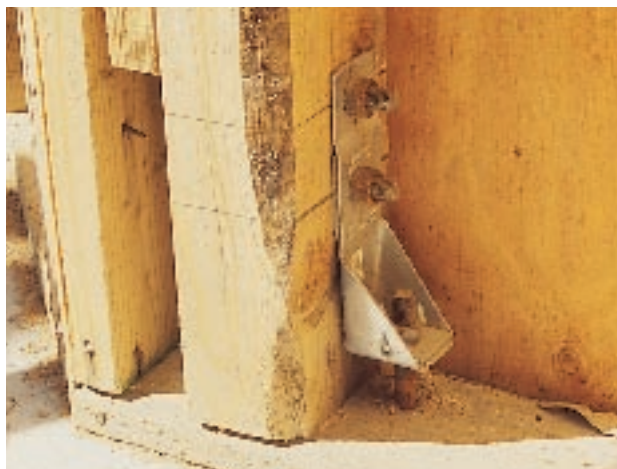
Figure 4. Some hold-downs, depending on the manufacturer, have to be held up a specified “standoff” distance from the plate, to ensure that the horizontal bolts don't tear out the end grain of the post under load.
