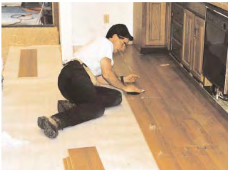
Figure 3. For hardwood strip flooring over radiant heating, always use a moisture barrier like Moistop (top), a fiber-reinforced composite of poly and Kraft paper popular with flooring contractors in the author’s area. Under floating hardwood floors, a pad like AstroBarrier (above) provides a foam cleavage layer and a poly moisture break.
