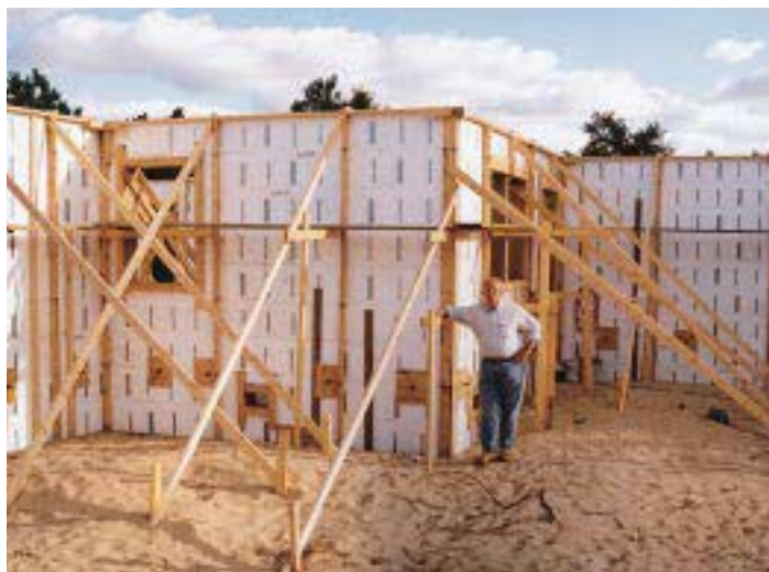
Spray foam dispensed from a can (left) glues the blocks together as they are stacked. Two-by-four bracing holds everything in place for the pour (right). Note also the squares of plywood holding the anchor bolts for the ledger in place.
