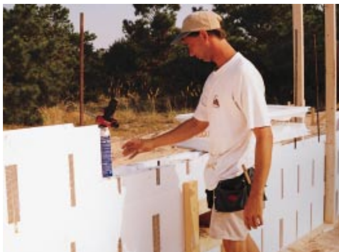
Spray foam dispensed from a can (left) glues the blocks together as they are stacked. Two-by-four bracing holds everything in place for the pour (right). Note also the squares of plywood holding the anchor bolts for the ledger in place.
