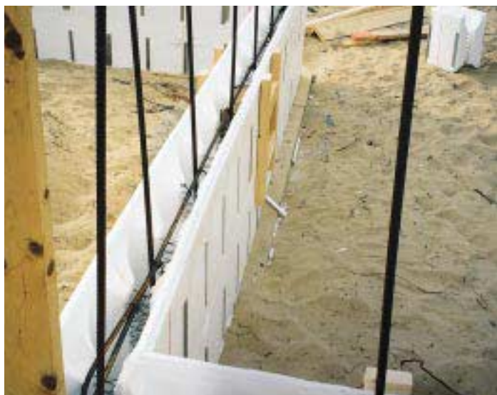
Vertical rebar, epoxied into place, extends from the footing (left) up through the Polysteel blocks. Horizontal rebar, laid in every other course, rests on the steel mesh that joins the sides of the blocks together, and is tied to the vertical rebar (right).
