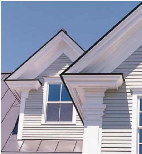
Figure 5. The finished return and the completed house. Note how the cornice details on the dormer have been scaled down.
