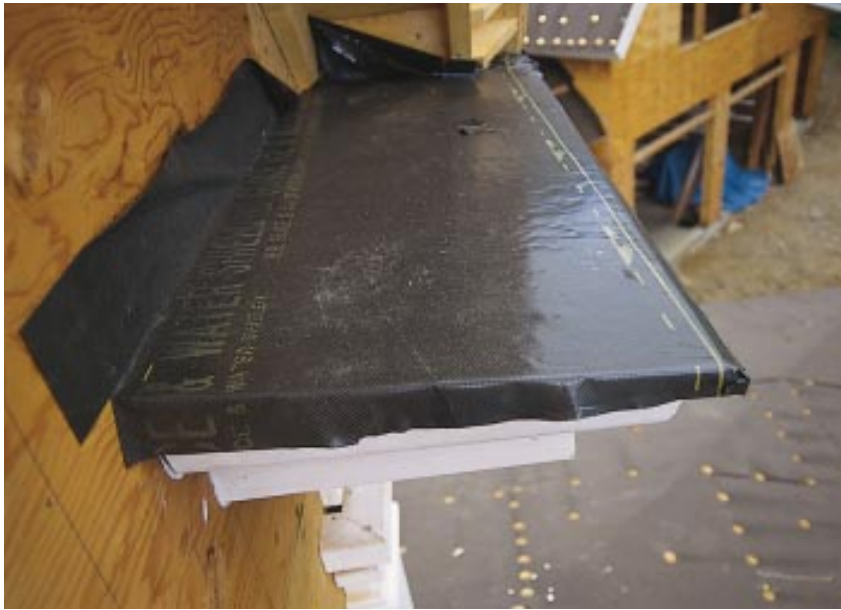
Figure 4. Eaves membrane protects the finished returns (above) until metal flashing is installed (right).
