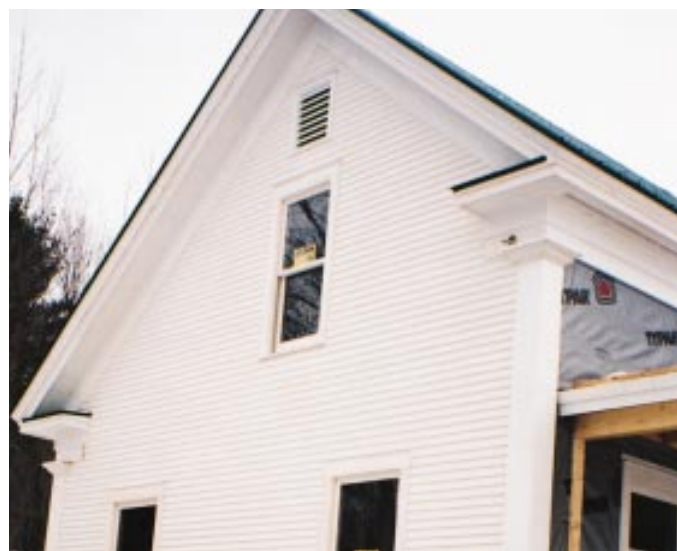
Figure 1. A simplified Greek Revival style cornice treatment uses flat stock with beveled edges — “poor man’s cove” — instead of a crown molding. Using flat stock makes it easy to turn the corner where the eaves meets the rake.
