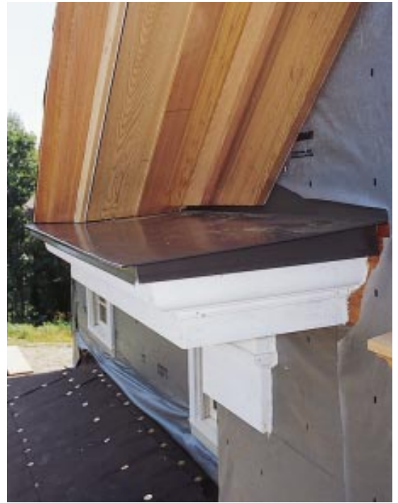
Figure 4. Eaves membrane protects the finished returns (above) until metal flashing is installed (right).
