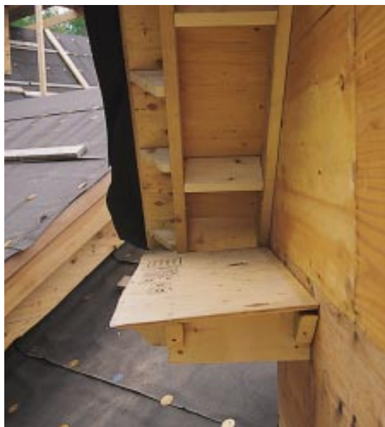
Figure 3. Angled blocks fastened with galvanized screws support the crown on the returns and up the rake (top). A plywood lid caps the return (left).
