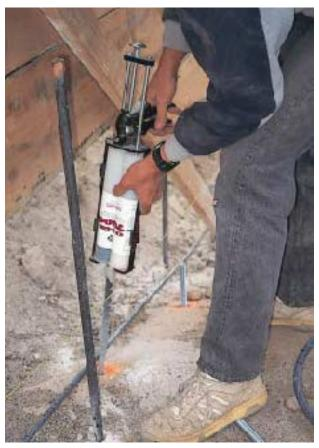
Dispensing adhesives. True epoxy-based adhesives are unaffected by water, making them a good choice for damp locations, such as foundation pins in water-bearing granite.
