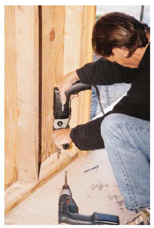
ial and the strength of bond, but also on the strength of the concrete or masonry. Ultimate shear loads give a measure of an anchor's resistance to forces across the face of the concrete or masonry — a force threatening to tear the anchor, and to crush the bearing material around the anchor.
