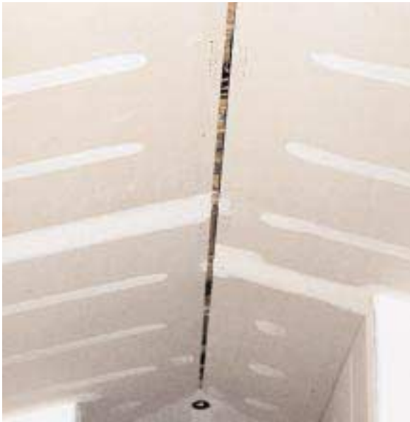
Figure 3. Gaps in drywall joints, like these at the peak of a cathedral ceiling (left), can cause bubbles or wrinkles in ordinary paper tape. UltraFlex's plastic backing not only bridges these kinds of gaps, but makes it easy to get a clean crisp line at the joint (right).
