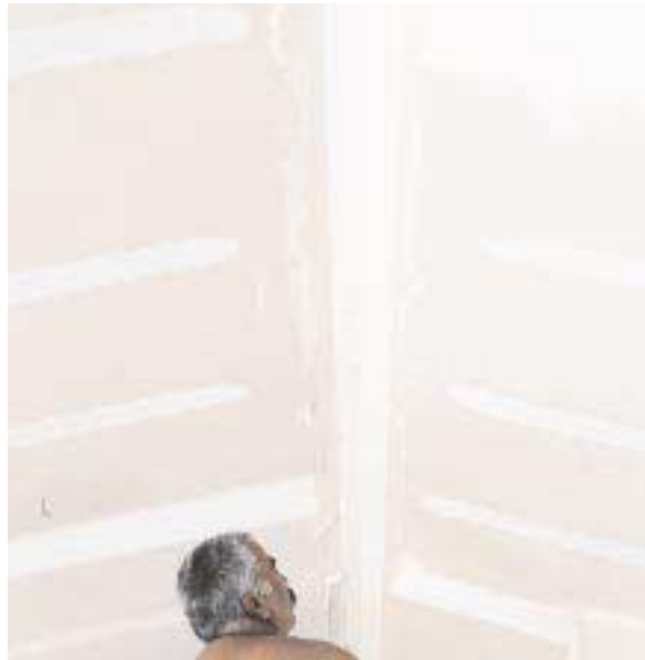
Figure 3. Gaps in drywall joints, like these at the peak of a cathedral ceiling (left), can cause bubbles or wrinkles in ordinary paper tape. UltraFlex's plastic backing not only bridges these kinds of gaps, but makes it easy to get a clean crisp line at the joint (right).
