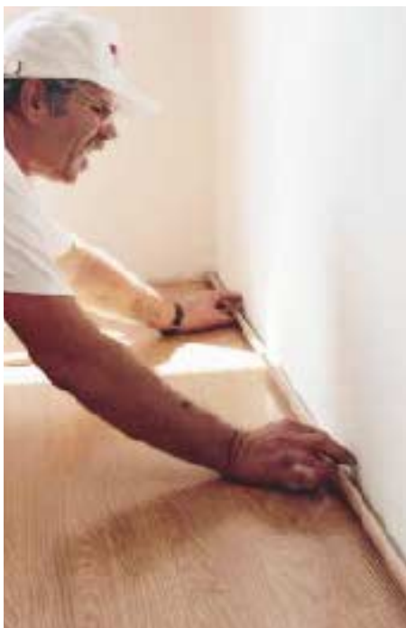
Figure 8. Careful undercuts at door jambs and casings make for a clean finish detail (above). At transition moldings, such as where laminate flooring meets tile and when installing base moldings (left), avoid getting any adhesive on the flooring or driving nails through the molding into the flooring. If floor movement is restricted in any way, seasonal dimensional changes can cause serious damage.
