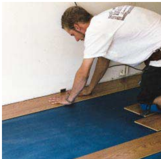
Figure 5. Use spacers (supplied by some manufacturers) or flooring scraps to establish the expansion gap. Note the blue foam underlayment.
