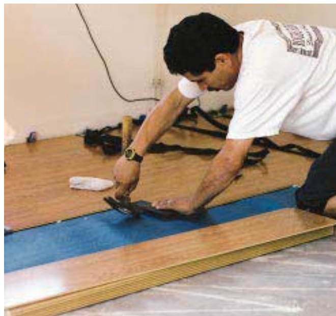
Figure 6. Using a tapping block, seat the end joints until an even glue line squeezes out. Most manufacturers supply strap clamps to hold successive courses in place until the glue dries. Staggered butt joints help to make the finished floor appear seamless.
