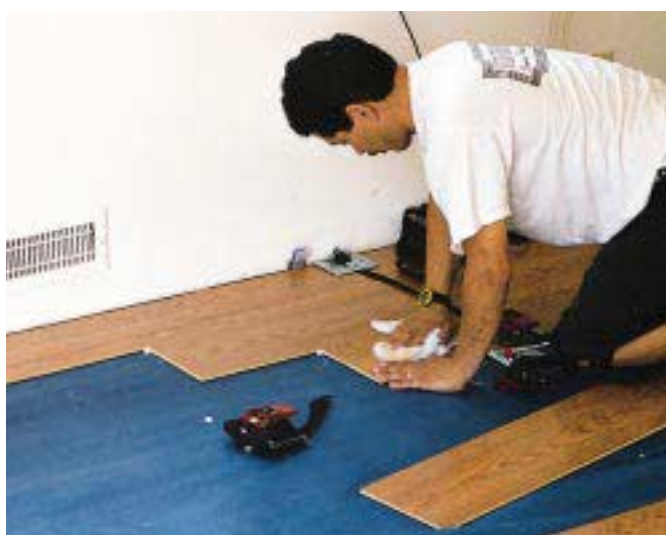
Figure 7. Some manufacturers recommend cleaning up the glue immediately; others advise allowing the squeeze-out to set up partially, then scraping it off.
