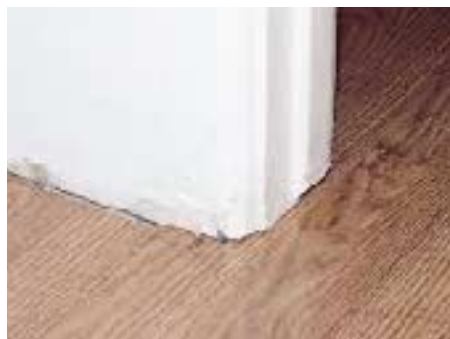
Figure 8. Careful undercuts at door jambs and casings make for a clean finish detail (above). At transition moldings, such as where laminate flooring meets tile and when installing base moldings (left), avoid getting any adhesive on the flooring or driving nails through the molding into the flooring. If floor movement is restricted in any way, seasonal dimensional changes can cause serious damage.
