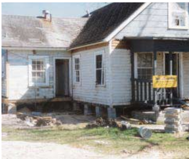
Figure 2. After decades of settling into the ground, this house (top) is showing serious moisture damage. New floor joists (middle) provide a sound structure for jacking. The framing nailed to the wall helps to pick up individual studs and the corner post. Note the new elevation of the porch rail relative to the concrete porch (bottom) as the house comes up.
