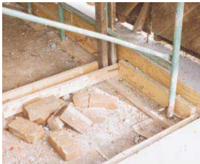
Figure 4. Staging made a convenient platform for jacking the carriage house (top), but it had to be thoroughly braced all the way to the ground. In addition to continuous cross-bracing in both directions, the author set 6x6 posts under the critical jacking points (middle), and made stable bases for the scaffold legs (bottom) by drilling holes in 2x6s.
