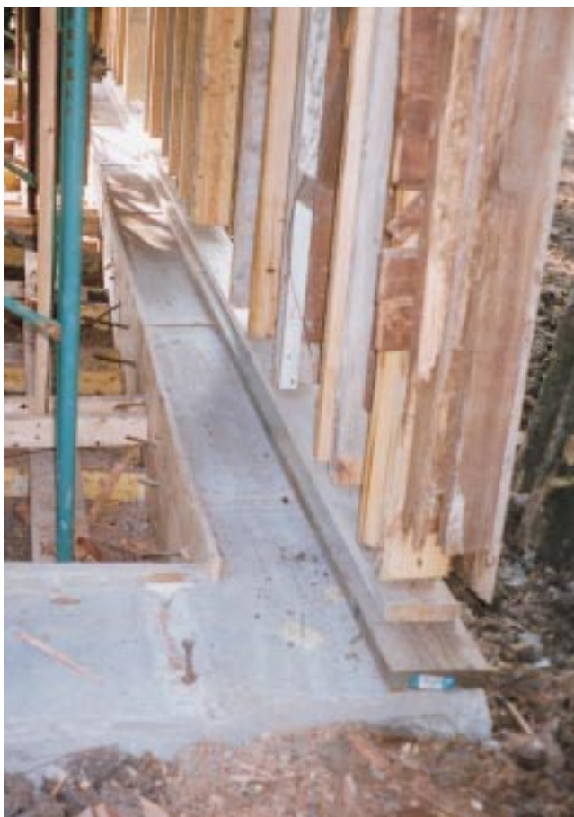
Figure 5. While the second story of the carriage house was suspended, the crew excavated, formed, and poured new footings (top), then repaired the wall framing and lowered the building onto new PT sills.
