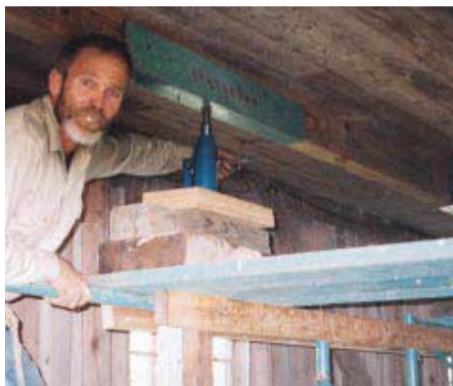
Figure 1. The author uses three types of jacks (from left in top photo): hydraulic, screw, and hypoid gear. Steel angle slips, predrilled for attaching with duplex nails, spread the load over a larger bearing surface (bottom photo).
