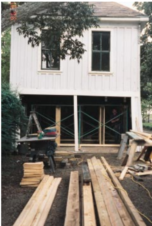
Figure 3. This turn-of-the-century carriage house was 19 inches out of level and 12 inches out of plumb before renovation. Termites had made mincemeat of much of its wall framing.
