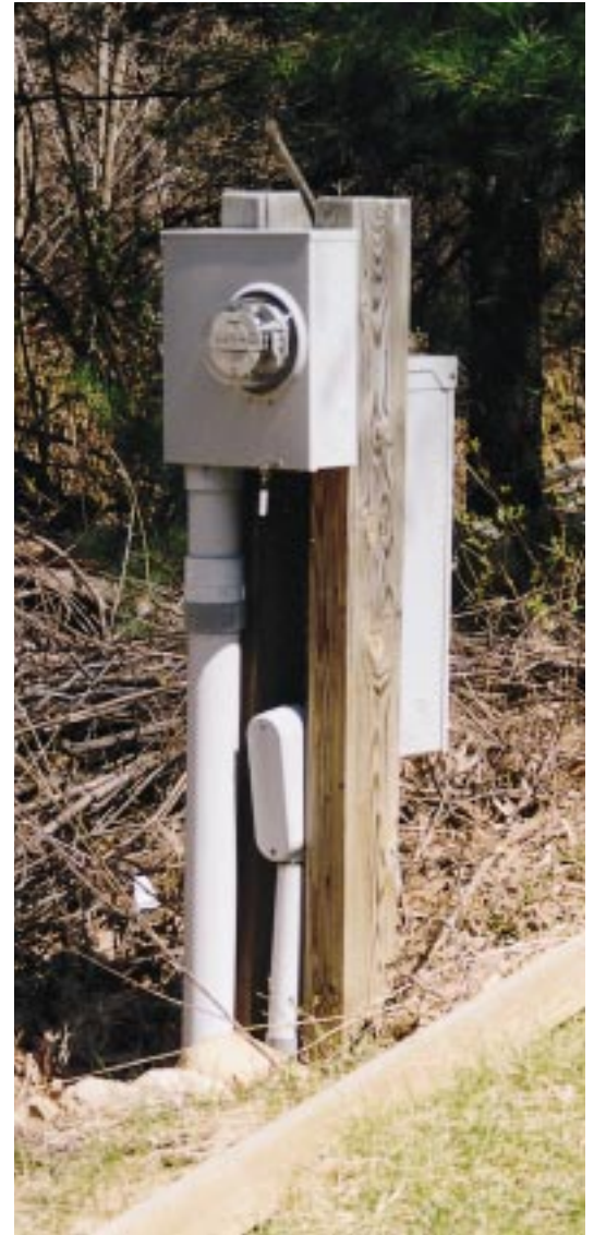
Figure 1. You may be able to install permanent power at the beginning of a job using a pedestal. The meter and main disconnect are installed on a short permanent post, while the power cable runs underground to the house service panel. If the panel is planned for the basement, you can install it immediately after the foundation forms are stripped. A pedestal is more expensive than overhead service, but you save the temporary hookup charge.
