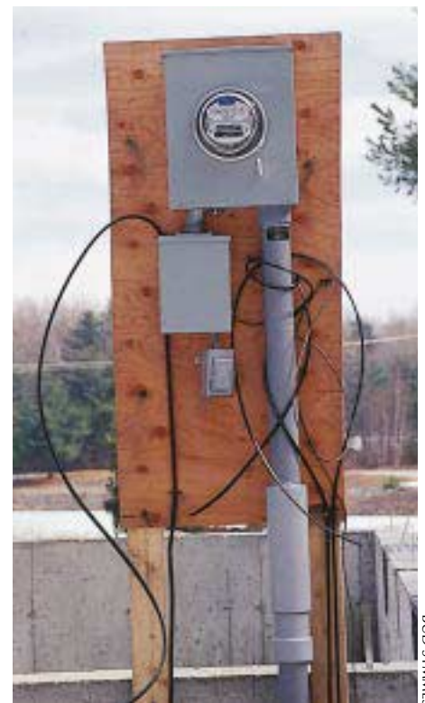
Figure 3. The meter socket, breaker panel, and GFCI receptacle on a temporary service must all be weatherproof (left). Overhead service requires a well-braced pole to support the mast (middle); underground service components should be temporarily mounted to a sturdy frame (right). Requirements vary, so check with your local utility for complete specs.
