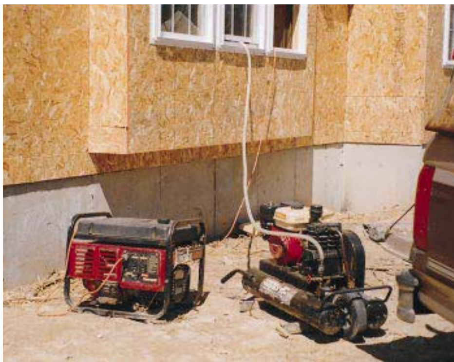
Figure 2. Generators save the temporary service charge, but they're noisy and you'll lose time gassing up and starting the engine on cold mornings. Depending on the size and number of power tools you use, you may also need a gas compressor, since a generator may not be able to supply enough amperage for an electric compressor.
