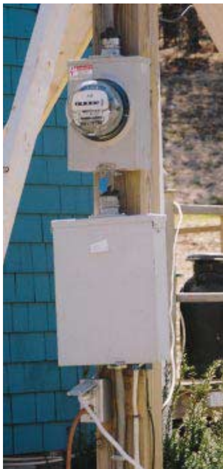
Figure 3. The meter socket, breaker panel, and GFCI receptacle on a temporary service must all be weatherproof (left). Overhead service requires a well-braced pole to support the mast (middle); underground service components should be temporarily mounted to a sturdy frame (right). Requirements vary, so check with your local utility for complete specs.
