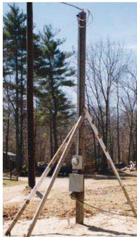
Figure 3. The meter socket, breaker panel, and GFCI receptacle on a temporary service must all be weatherproof (left). Overhead service requires a well-braced pole to support the mast (middle); underground service components should be temporarily mounted to a sturdy frame (right). Requirements vary, so check with your local utility for complete specs.
