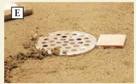
protruding from the drain, and press the membrane over all four bolts. Finally, I snug down the bolts and cut a hole in the membrane to open the pan to the drain.
