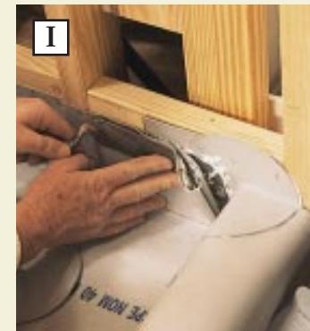
difficult to work with and prone to leaks. For the past 20 years, I've been using chlorinated polyethylene (CPE) sheet membrane to fabricate pan liners for showers, sunken tubs, fountains, and other wet tile installations. Available from the Noble Co. (614 Monroe St., Grand Haven, MI 49417; 616/842-7844), CPE membrane, called Chloraloy, comes in 4-, 5-, and 6-foot-wide rolls, and can be bonded to itself to make shower pans of any size.
