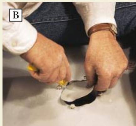
To fit the membrane around the clamping drain, first cut small holes for the flange bolts (A) and push the membrane over the protruding bolts. Then slice the membrane around the inside diameter of the drain (B) before bolting the clamp ring in place (C) and adjusting the finish drain stem to the proper height (D). To prevent mortar from plugging the drain's weep holes, circle the drain with plastic tile spacers (E).
