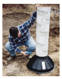
and the form can be left in place after the pour. The flared design shapes a smooth, coneshaped footer on the pier, and you can even turn a spare form upside down and use it as a funnel while pouring mud into the other forms. Bigfoot has been spotted in most areas for about \$15 each.
