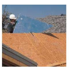
turer as a "radiant barrier overlay," TechShield looks a lot like aluminum foil. It's laminated to a sheet of gradestamped plywood or strand board, then perforated so the substrate can breathe. Nail this product off just like you would any sheathing, but make sure the foil
