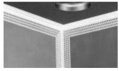
beads are bedded in joint compound rather than fastened with nails or screws, then topped with a finish coat after the base dries. Where time is tight, you can staple the bead in place and apply the finish coat immediately.
