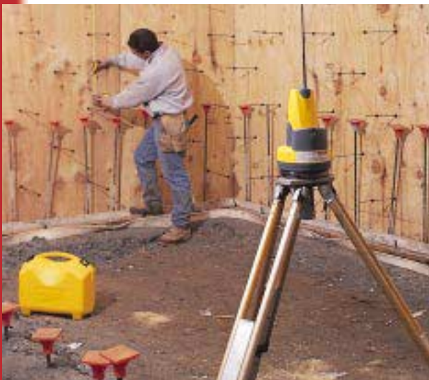
Figure 6. Moveable dot. The single laser dot emitted by a self-leveling RoboLaser can be moved to any position with a hand-held remote. While the machine turns slowly, the dot tends to be much easier to locate than the dim line made by the spinning dot from a rotary machine.
