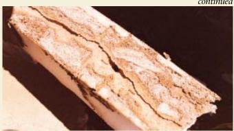
David Damroth discovered the extent of a termite infestation in his home by removing a 6-inch band of insulation from the perimeter of the foundation (left). He found a dense network of termite shelter tubes behind the foam, as well as along the top of the foam (right), where the bugs had traveled around the house looking for a point of entry.
