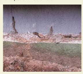
The termites were hidden from view by the foam, through which they carved numerous tunnels (left). They eventually entered the house between overlapped layers in the copper termite shield at the house corners; in some cases, they built shelter tubes around the termite shield (middle). Damroth removed the tubes, but within hours, the termites had begun to build new tubes (right).
