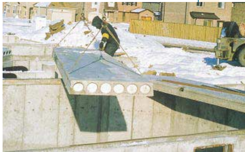
Figure D. These precast concrete panels are fabricated with hollow cylindrical cores that can be used to run wiring and piping. Installation is typically handled by special crews using a crane or boom truck.
