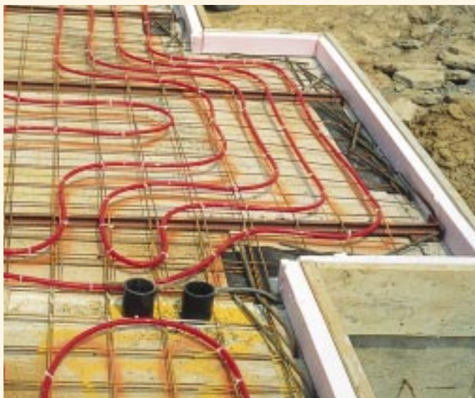
Figure 4. When laying radiant floor heat tubing, lines snapped directly on the plywood forms help installers to avoid interior partitions. The tubing is laid on top of and tied to welded wire mesh.
