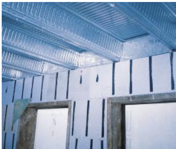
Figure B. Both shallow-pan (left) and deep-pan forms (above) are available. With temporary supports removed, the concrete-and-steel "composite" deck can span long dimensions and leaves a clean appearance on the underside.
