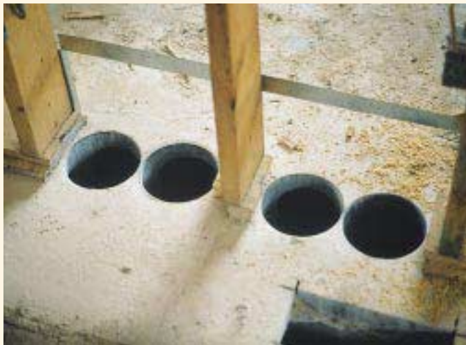
Figure 3. Openings for electrical and mechanical systems are blocked out with empty paint cans or cut with a concrete saw. Stairwells and other large rough openings are blocked out with 2x4s fastened to the plywood forms.
