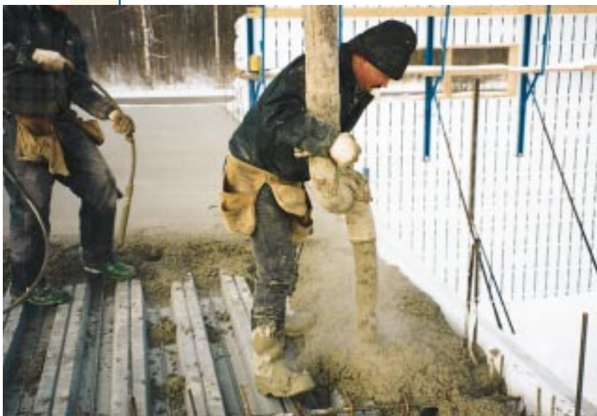
Figure A. Thorough vibrating during the pour ensures a good bond between slab concrete and the steel pan forms.
