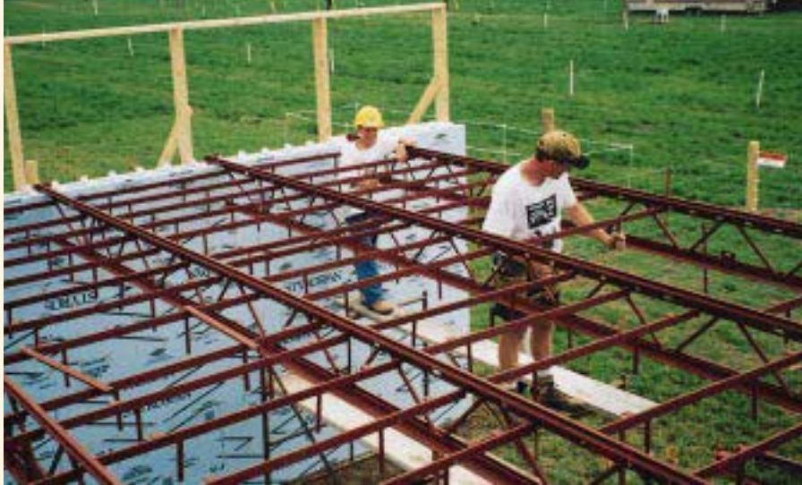
Figure 1. To ensure that the plywood forms will interlock properly, each Hambro joist is tagged to match markings on the working drawings provided by the manufacturer. Reusable steel rollbars automatically set the on-center joist spacing. A two-man crew can form a 2,000-square-foot slab in 10 hours.
