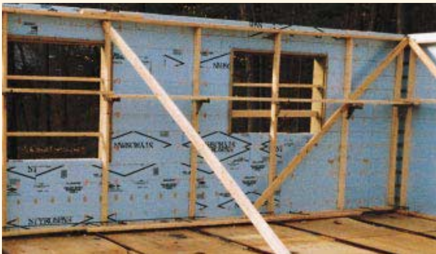
Figure 2. Interior partition locations are snapped directly on the plywood forms prior to installing radiant heat tubing and blocking out other mechanicals. Here, the plywood is also being used to brace second-story ICFs.
