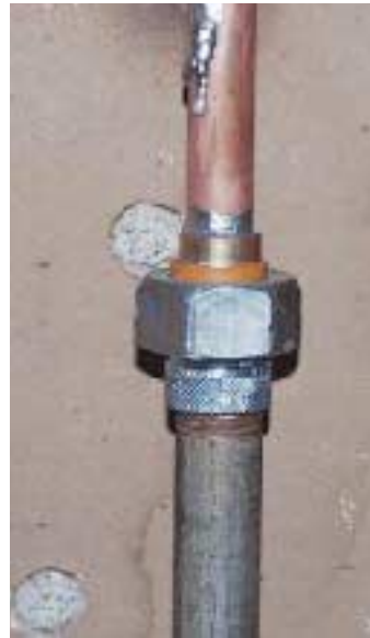
Figure 5. A dielectric union makes it possible to join new copper to existing galvanized pipes without the risk of galvanic corrosion.
