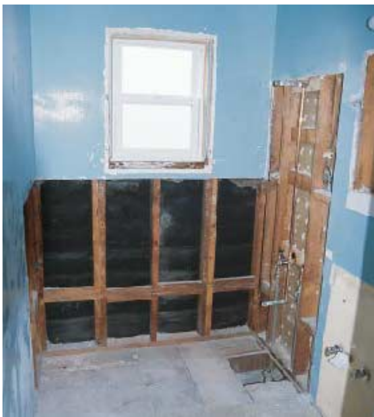
Figure 4. The crew keeps demolition to a minimum, removing only as much plaster as absolutely necessary (above). To avoid having to match new fixtures to old plumbing, the author replaces all supplies, valves, and traps (top).
