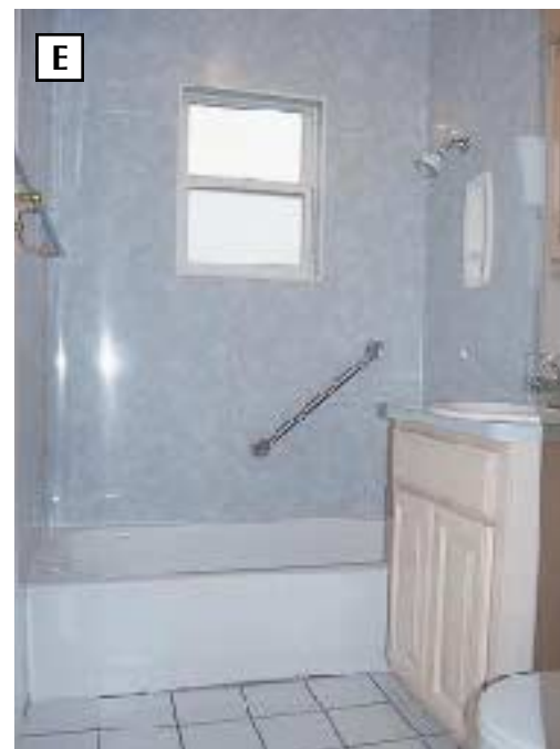
Figure 6. The last day of the four-day bath remodel is a busy one: The shower surround is installed and trimmed (A), light fixtures and cabinets are hung (B & C), the tile is laid, and the toilet and vanity are set (D & E). After final trimming out, the crew leaves the homeowners with a warning to stay off the floor until the grout cures.
