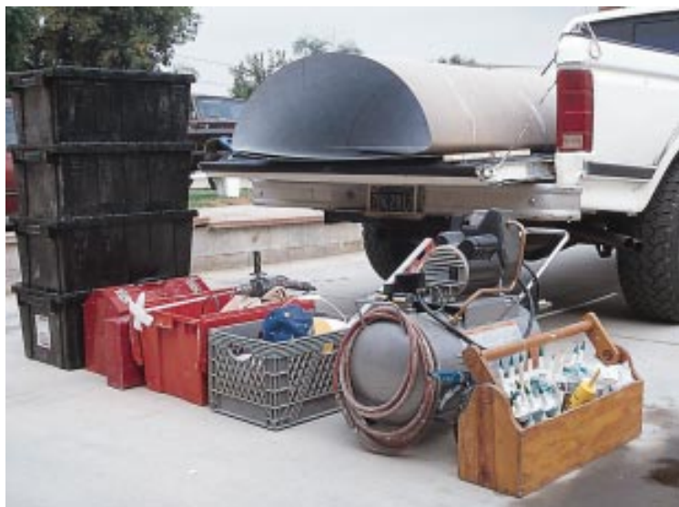
Figure 3. All the tools and materials needed for the fast bath remodel are organized using a system of crates and bins.
