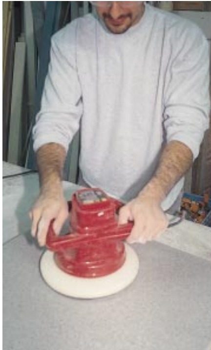
Figure 6. All Swanstone seams and edges are sanded with an orbital sander. Finally, the surface is polished with a rubbing compound.
