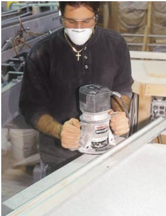
Figure 2. At seams, the author insets a 1½-inch-wide Swanstone strip into a dado in the substrate (left). This provides reinforcement to the butt joint. To ensure tight seams, butting edges are routed with a straight-edge (right).
