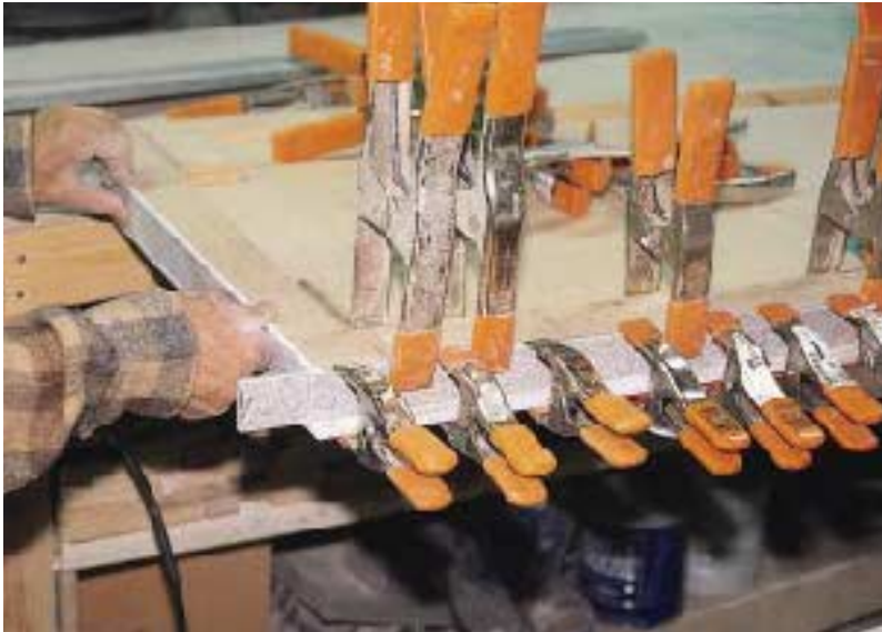
Figure 4. With the top flipped upside down, the edge banding is attached with acrylic adhesive and spring clamps (above). The edging fits tight against the bottom of the overhanging top surface. After the glue sets, the counter is flipped over and the top is routed flush with the edging.
