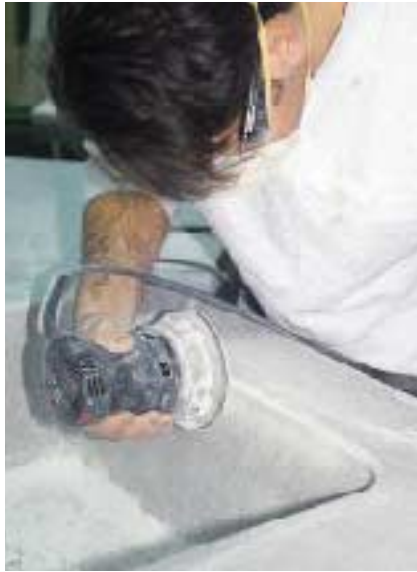
Figure 6. All Swanstone seams and edges are sanded with an orbital sander. Finally, the surface is polished with a rubbing compound.
