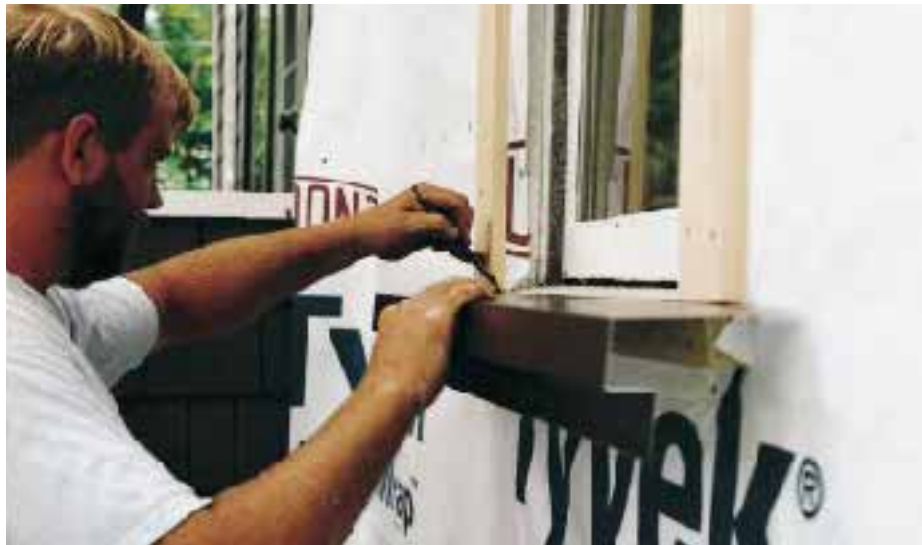
Figure 3. The author begins at the sill, scribing the brake-bent metal to finish length (above), then cutting returns with tin snips (left). Trim is never nailed through the face. Instead, fasteners are driven through the flanges and tabs (below), which are planned carefully so that joints drain properly without relying on caulk.
