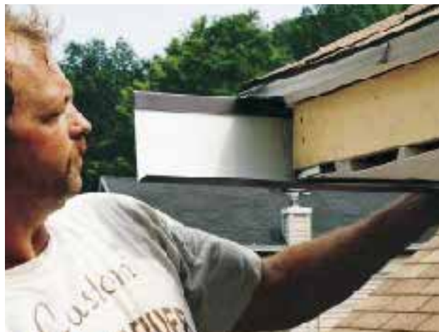
Figure 5. To prevent buckling, the hemmed upper edge of the fascia trim metal is tucked under the existing drip edge, and nailed up from the bottom through the soffit (left). Similarly, the trim is allowed to “float” when covering old fascia molding (see illustration). To cover two-piece fascia, or when the roofline dips and sags, use two-piece trim nailed up from the bottom only.
