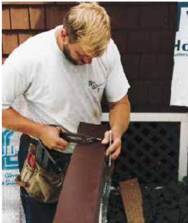
Figure 3. The author begins at the sill, scribing the brake-bent metal to finish length (above), then cutting returns with tin snips (left). Trim is never nailed through the face. Instead, fasteners are driven through the flanges and tabs (below), which are planned carefully so that joints drain properly without relying on caulk.
