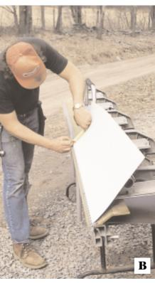
After marking a centerline on the valley flashing, the author forms the ridge of the V-crimp (A). A layout line representing one side of V-crimp base is marked 1 inch from the centerline fold (B). The flashing is flipped upside down, reinserted in the brake, and bent at the layout line (C, next page). After turning the flashing around in the brake, the opposite V-crimp base is folded (D).
