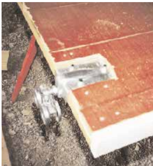
Figure 7. Metal mending plates reinforce the connections on 2x4 sliding door frames (above). Off-the-shelf hardware is concealed by decorative 1-by trim (left).
