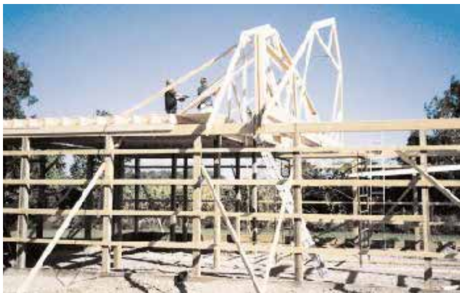
Figure 5. Building the second-floor deck at the rear of the building first provided a work area for raising storage trusses over the front half of the barn (above). The joints in the two-piece site-built gambrel rafters were supported by triple-2x8 headers; second-floor posts bear directly over posts below (left).
