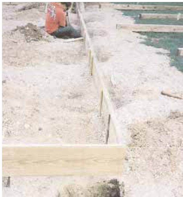
Figure 1. Batter boards and string guide the layout, and form stakes keep the grade board aligned. Temporary wood shims holding the grade board at the proper elevation were replaced later with crushed stone.
