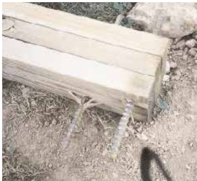
Figure 2. To resist uplift, short lengths of rebar were driven through holes drilled in the bottom of the posts.
