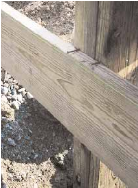
Figure 3. Prior to pouring the concrete, each perimeter post was diagonally braced to grade stakes and suspended over its post hole by a pair of 16-penny nails resting on top of the grade board (right). The four center posts were held at the proper elevation by nail-on cross-tees, and tied to the outside posts with lateral bracing (bottom).
