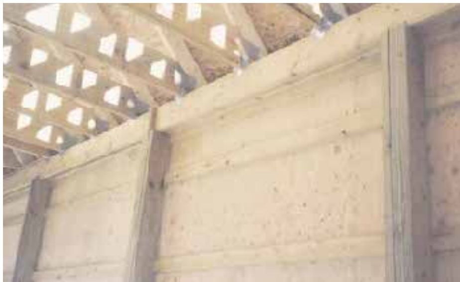
Figure 4. The triple-2x8 perimeter headers were supported by full posts at midspan, and by a shoulder at each end, created by cutting short the outside 2x6 on every other post.
