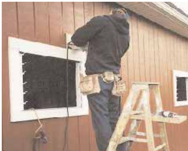
Figure 6. The author uses the head trim to guide a plunge-cut kerf in the T1-11 siding (right). Custom-bent flashing fits into the kerf above windows and the sliding-door track valance shown here (middle), and is held in place and sealed with paintable rubberized caulk (bottom).
