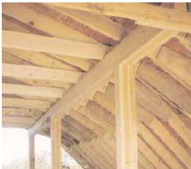
Figure 5. Building the second-floor deck at the rear of the building first provided a work area for raising storage trusses over the front half of the barn (above). The joints in the two-piece site-built gambrel rafters were supported by triple-2x8 headers; second-floor posts bear directly over posts below (left).
