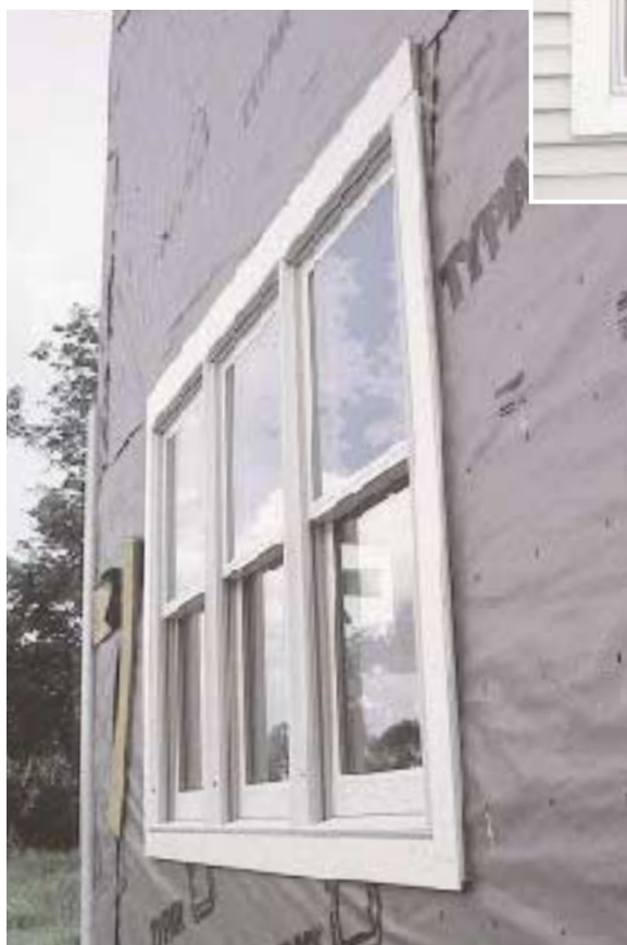
Figure 1. To avoid exposed J-mold, the author conceals the ends of vinyl siding behind a rabbet cut into the outside edges of 5/4 pine trim. To protect against moisture, the window flanges are set in silicone caulk over a layer of bituminous membrane or felt that rims the opening.
