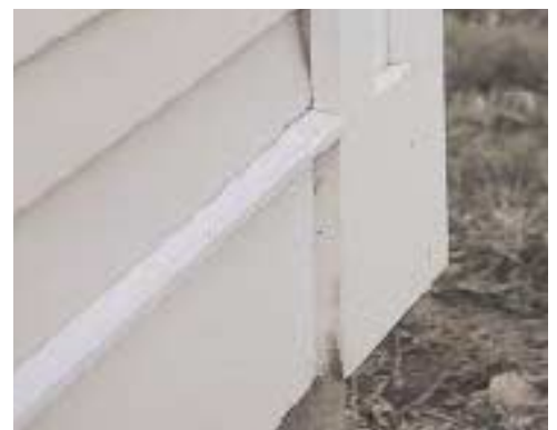
Figure 3. At corners, the rabbet conceals the ends of the vinyl siding and provides good drainage at the vertical joint where the corner trim passes by the skirt board (top). At built-up cornerboards, 1-by stock applied over spacers achieves the same clean look (above).
