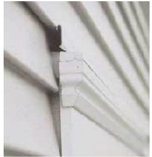
Figure 2. J-mold is exposed only above the head trim (photo). The molding is cut long and the ends are turned down to direct runoff into the rabbet. At the sill trim, a piece of vinyl undersill trim holds the vinyl siding in place (illustration, left).
