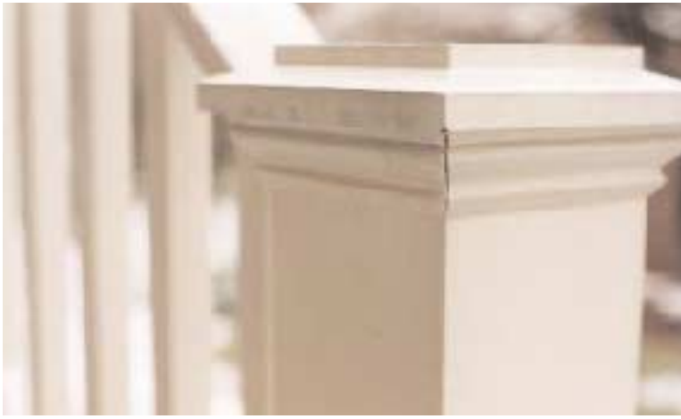
Figure 1. Miter joints stay tight only when temperature and humidity match the day they were installed. When the weather changes, miters tend to open up and allow water to get in and cause rot.
