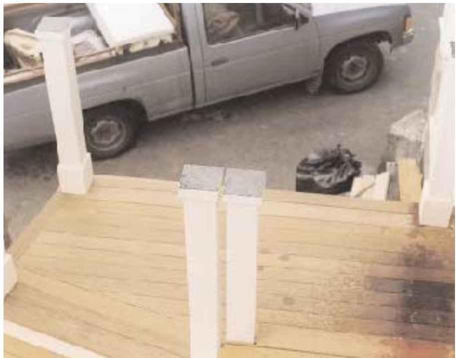
Figure 9. Nail-free decking systems can dress up a job and reduce points of water penetration. Notice how the author's crew flashes off the newel tops before installing caps.
