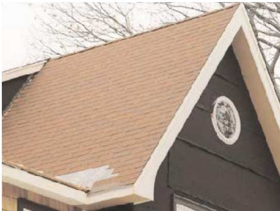
Figure 3. The deep eaves on this remodel give extra protection to walls and windows beneath.
