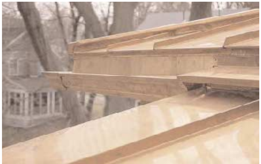
Figure 5. Properly flashed gutters keep water out from between the gutter and fascia boards. Gutters should also be cleaned frequently to prevent clogging and overflow.
