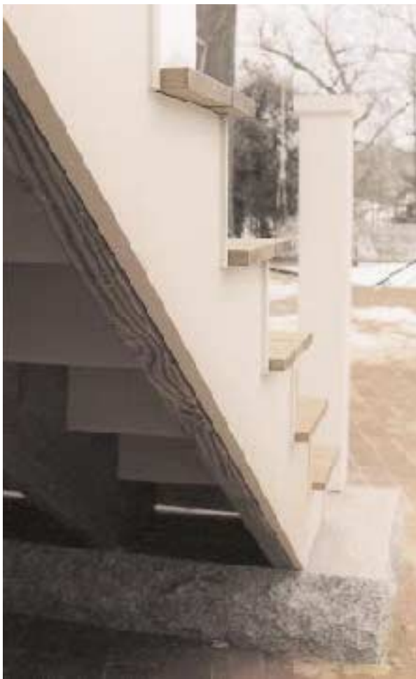
Figure 2. Avoid miter joints on porch and deck stair trim. Instead, run stair risers long and butt the skirt board into the risers.
