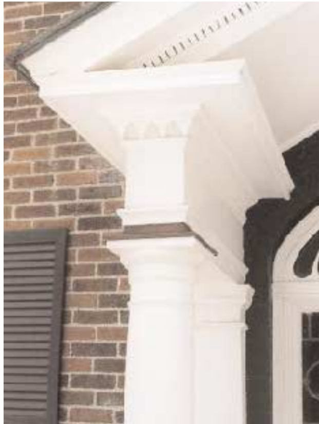
Figure 8. Flat surfaces are especially susceptible to water damage and require taking special precautions. On this porch, the column cap is completely capped with metal flashing, and the decorative trim above is also extensively flashed.
