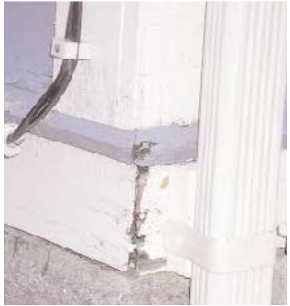
Figure 1. Miter joints stay tight only when temperature and humidity match the day they were installed. When the weather changes, miters tend to open up and allow water to get in and cause rot.
