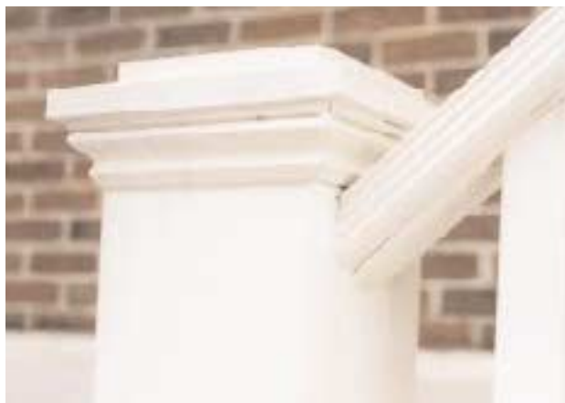
Figure 7. Prevent water penetration where rails join newels by adequately priming the end cut of a rail. It also helps to avoid rails that are wider than 5½ inches. When newels posts are wrapped, butt the rails directly against the trim instead of running rails through to the post where water will get trapped.
