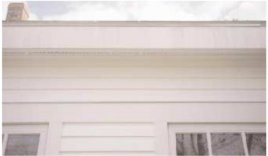
Figure 4. If drip edge is installed too close to the fascia, rain runoff will drain over the boards and lead to discoloration. The author recommends spacing drip edge slightly off of exterior trim to direct water outwards.
