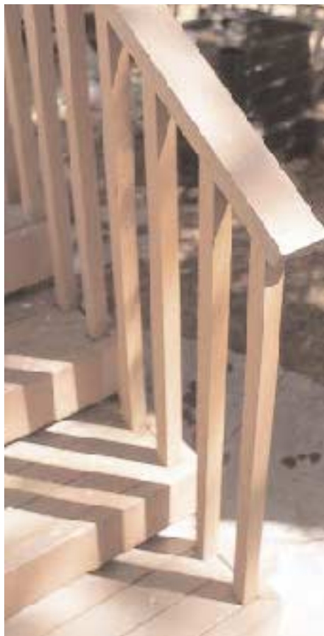
Figure 6. The bottoms of wooden porch and deck balusters are particularly prone to rot when they rest directly on a flat bottom rail. Besides always end dipping balusters, alternative designs can help — such as running balusters through the decking (left) or using a chamfered bottom rail that drains water (right).
