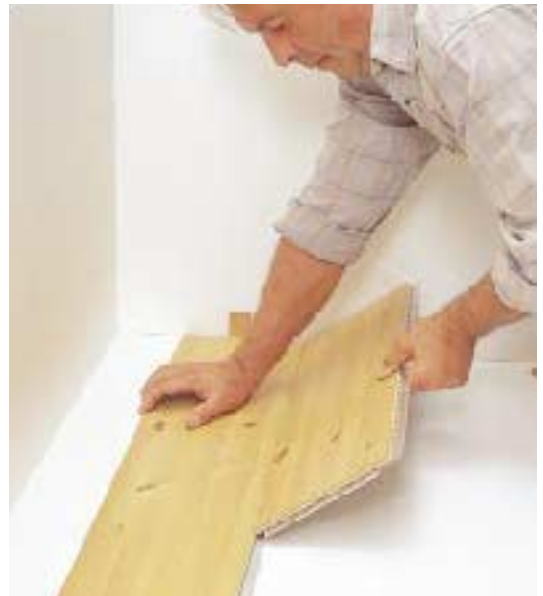
Figure 2. The Junckers solid-sawn flooring system is fastened with metal clips (left). Norske Skog’s Alloc flooring (above), uses an interlocking edge to hold planks together.
