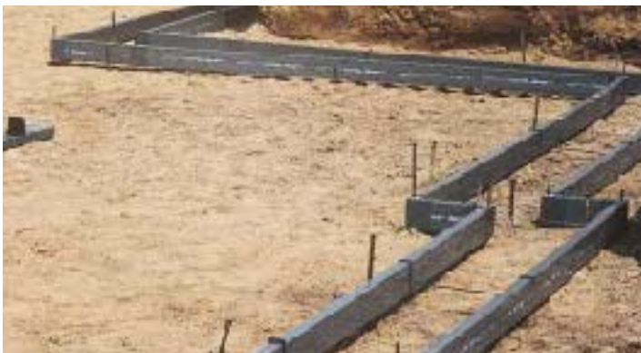
Figure 8. Form-A-Drain stay-in-place footing forms ensure a level perimeter drain and have a larger capacity than pipe systems (above). To control hydrostatic pressure, dimpled drainage panels fastened against the foundation wall carry water from the backfill into the perimeter drains (right).
