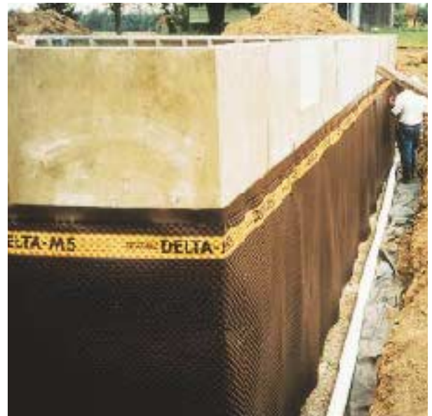
Figure 8. Form-A-Drain stay-in-place footing forms ensure a level perimeter drain and have a larger capacity than pipe systems (above). To control hydrostatic pressure, dimpled drainage panels fastened against the foundation wall carry water from the backfill into the perimeter drains (right).
