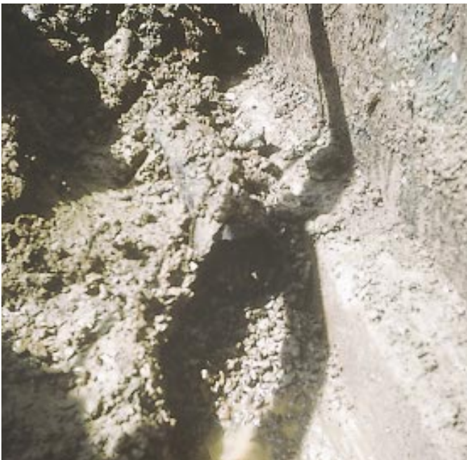
Figure 4. Without a filter to keep silt from contaminating the surrounding stone, drain tile can be rendered useless within just a few seasons (left). Pipe that is pre-wrapped or "socked" with filter material will prevent drain tile from becoming plugged (above).
