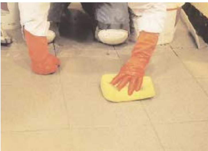
Figure 8. Begin cleaning by wiping the tile with a clean, damp sponge, using a light circular motion, then make a final pass with the sponge using long, straight strokes (above). After the tile dries, remove any grout haze from the surface with a soft cloth or towel (right).
