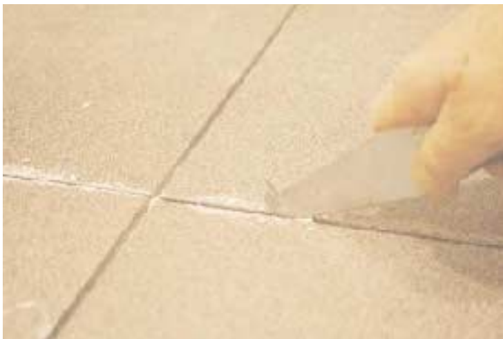
Figure 1. Patches of excess adhesive buildup in the joints can cause splotches on the surface of colored grout. If the adhesive hardens before it can be removed, cut away any excess with a tuck-pointing trowel or scraper to a depth of two-thirds the tile thickness.
