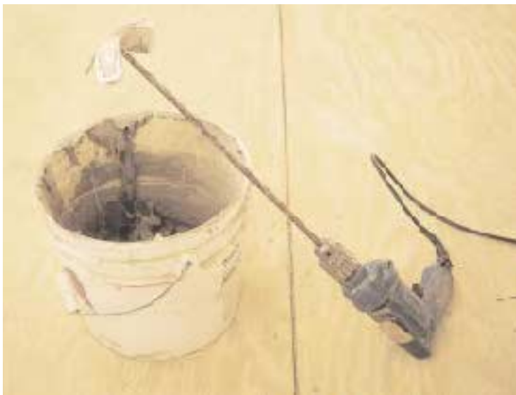
Figure 3. Grout is best mixed slowly by hand. For larger quantities, mix at slow speed with a paddle mixer chucked into a 1/2-inch drill. As the grout is applied, remix every five or ten minutes to keep the grout workable.
