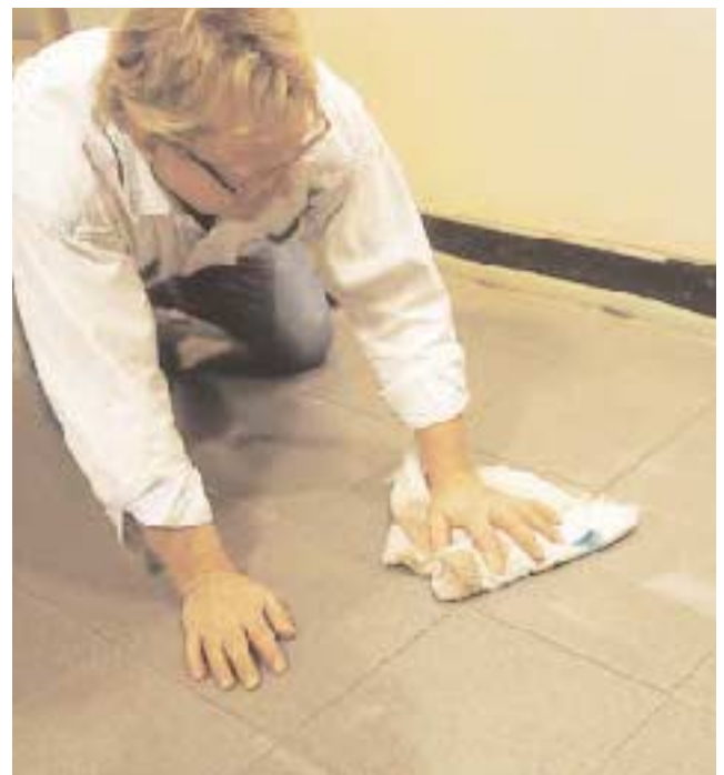
Figure 8. Begin cleaning by wiping the tile with a clean, damp sponge, using a light circular motion, then make a final pass with the sponge using long, straight strokes (above). After the tile dries, remove any grout haze from the surface with a soft cloth or towel (right).
