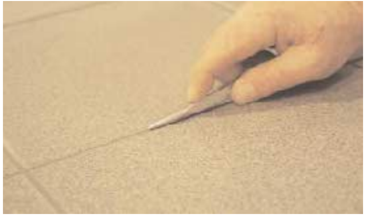
Figure 9. Sanded-grout joints on floors or countertops will be easier to keep clean if you push the sand particles below the surface by striking the joint with a nail set or dull drill bit.
