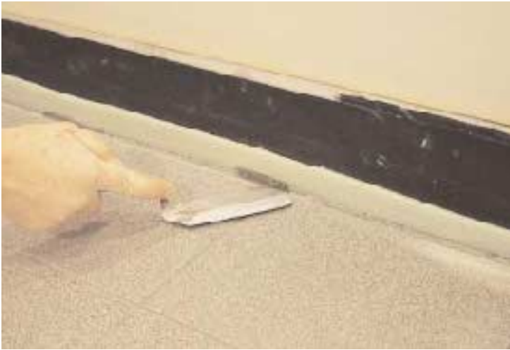
Figure 7. After the grout has begun to harden, use a dull knife or the tip of a trowel to slice it out of expansion joints, which will later be filled with caulk.
