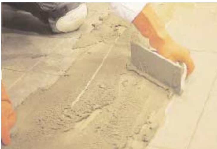
Figure 6. Force the grout into joints by holding the rubber trowel at a shallow angle as you sweep it over the tile from several directions (left). To scrape away the excess, hold the trowel on edge and stroke the surface on a diagonal to the joint direction (above).
