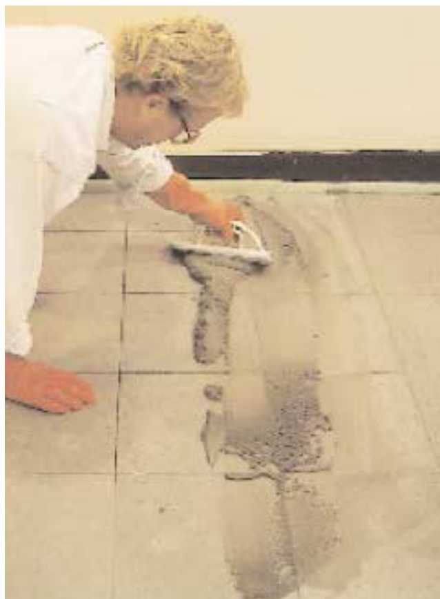
Figure 6. Force the grout into joints by holding the rubber trowel at a shallow angle as you sweep it over the tile from several directions (left). To scrape away the excess, hold the trowel on edge and stroke the surface on a diagonal to the joint direction (above).
