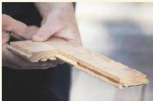
Figure B. The author makes splines to use whenever he has to run the flooring groove side to groove side.
