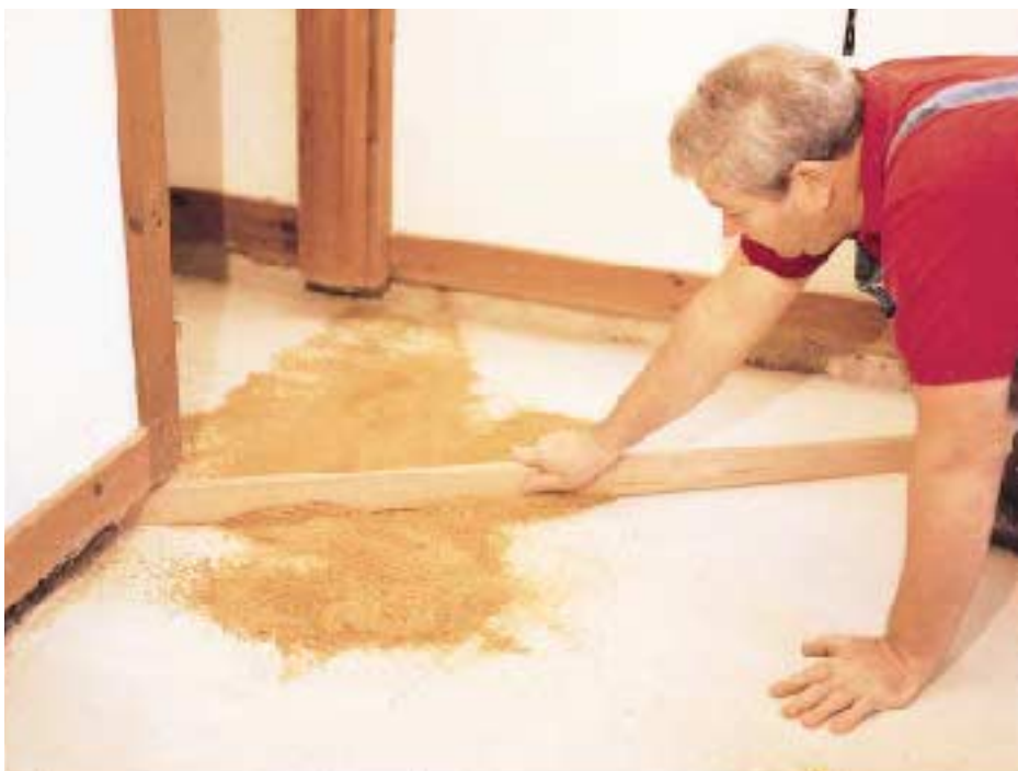
Figure 4. The author screeds dry mason's sand to level a low spot on a slab before installing a plywood nailing substrate. The trick with this technique is to avoid stepping in the sand after you've screeded it level and covered it with a poly vapor barrier.
