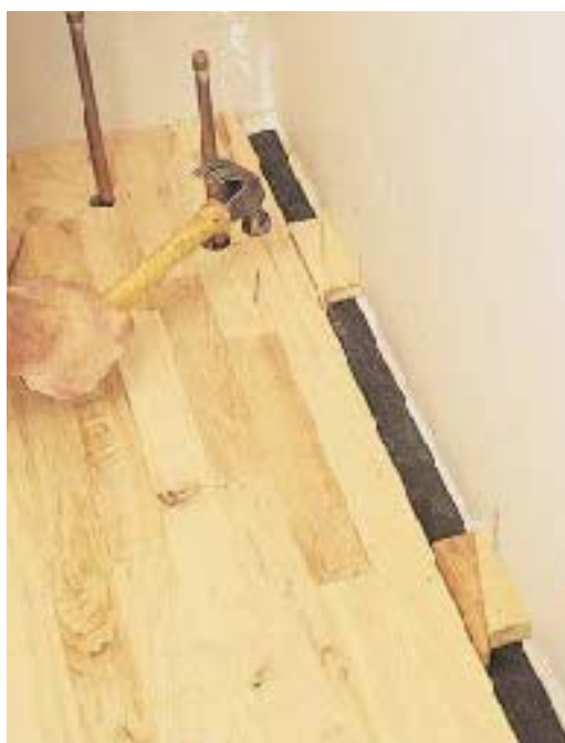
Figure 7. You need to drive lots of nails into wood flooring to hold it firmly in place during regular seasonal climate swings. The wider the flooring, the more nails that need to be driven along the nailing edge of each board.
