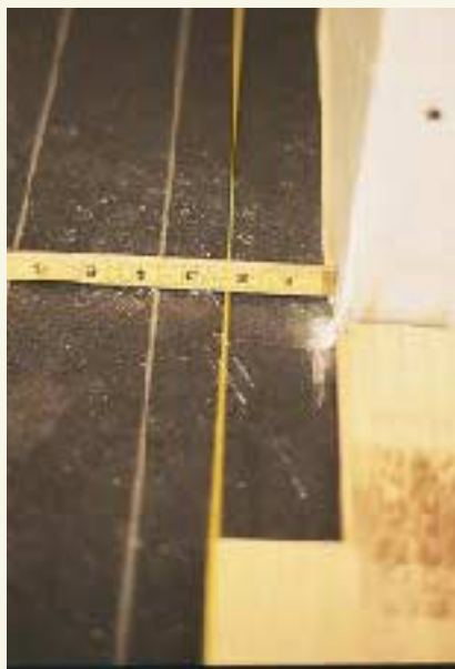
Figure A. Snapping a chalk line to start the layout in a new room ensures the flooring runs parallel to the walls.
