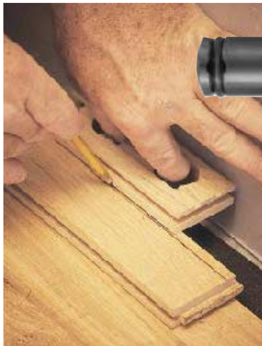
Figure 8. Because he uses plenty of nails to keep the flooring from moving, the author doesn't leave perimeter expansion spaces on typical residential strip flooring installations. Countersunk face nails hold the perimeter strips snug; the last strip is scribed tight to the wall. To prevent splitting when nailing these last courses, the author uses a nail spinner from Vermont American (inset), which chucks into a drill, to drive the finish nails.
