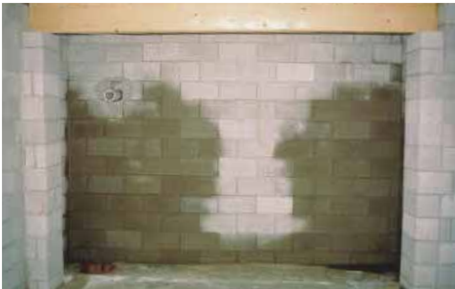
Figure 12. Omitting flashing and weepholes is risky. Water that penetrates brick veneer can saturate wood framing or enter the basement.
