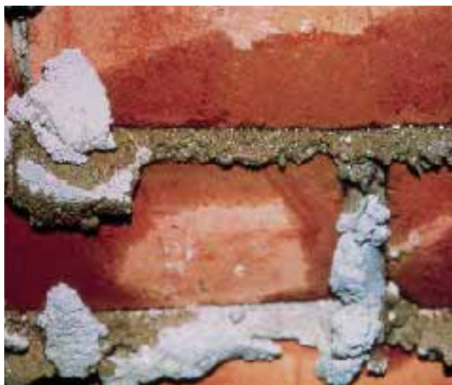
Figure 1. Since wind-driven rain may penetrate brick veneer, it is best to assume that the backs of the bricks will be wet. Unless the water can drain to the exterior, moisture can damage framing or interior finishes.
