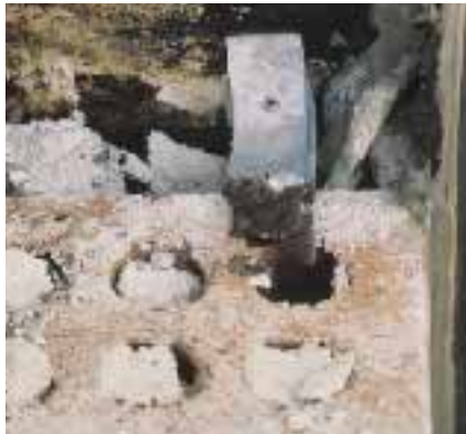
Poor workmanship and wind-driven rain may reduce the strength of masonry walls to levels below code. Corrosion of galvanized steel brick ties can also lead to failure.
