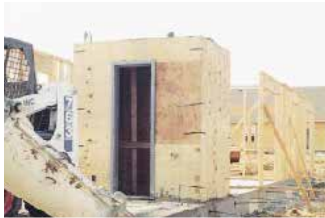
Poured concrete safe room under construction in Oklahoma.
