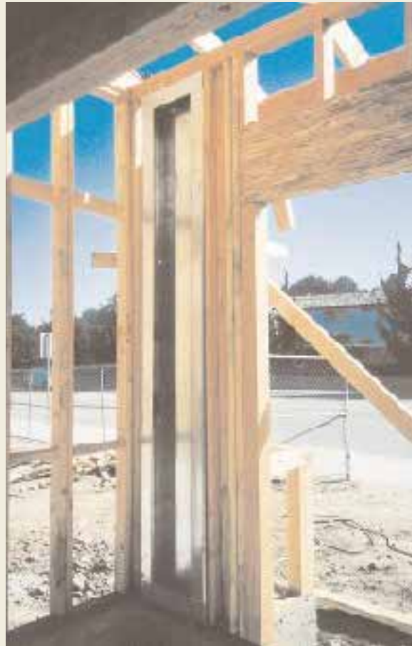
Hardy Frame is available as a narrow panel for use next to garage openings.
