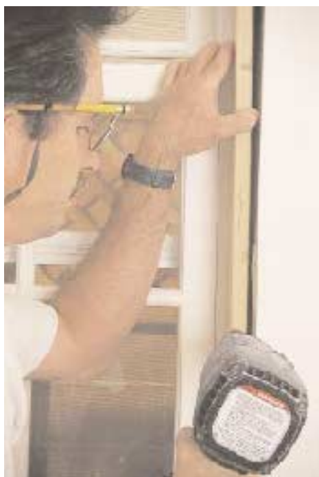
Figure 2. MDF is not a good material to use for extension jambs. While it mills easily and takes paints well, it tends to split when screwed or nailed through the edge.
