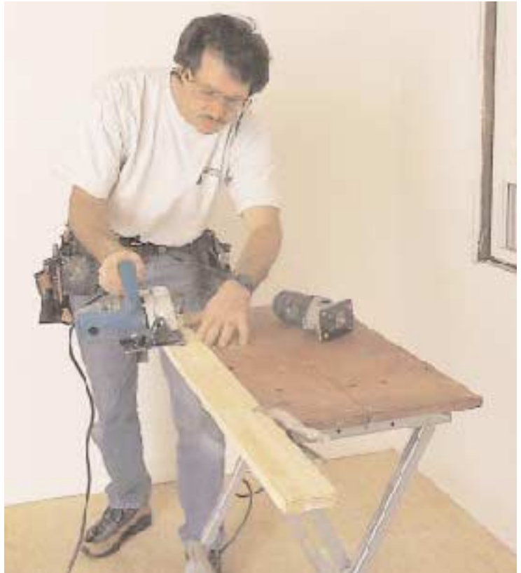
Figure 9. When the window is out of plane with the wall, paint-grade extensions can be individually scribed (above), then ripped with a panel saw and sanded (right). For stain-grade extensions, however, the author prefers to measure both ends of each piece to make sure the ends mate perfectly.
