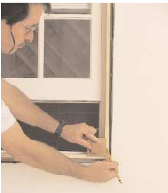
Figure 8. To achieve a consistent reveal when installing stacked extension frames, the author uses a wood block milled on all four edges.
