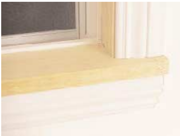
Figure 5. On windows trimmed with a stool and apron, the stool horns must be long enough to catch the casings (above). If the horns need to be scribed for a tight fit against the wall (above right), the author creates a slight back-cut using a panel saw (right).
