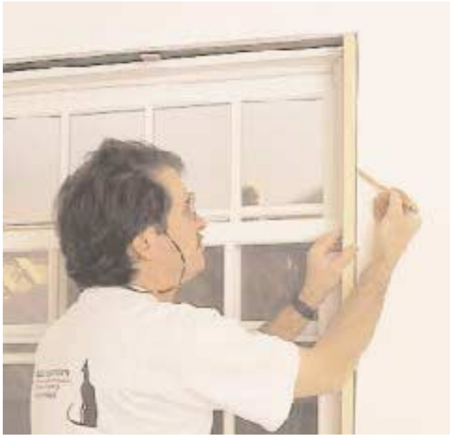
Figure 9. When the window is out of plane with the wall, paint-grade extensions can be individually scribed (above), then ripped with a panel saw and sanded (right). For stain-grade extensions, however, the author prefers to measure both ends of each piece to make sure the ends mate perfectly.
