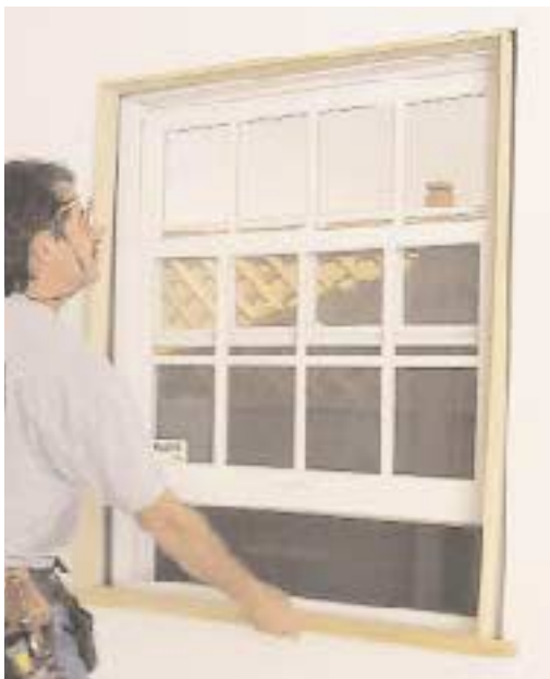
Figure 7. After positioning the preassembled frame against the window jambs (above), screw the extensions through the back-rabbets (above right), and fasten the stool through the countersunk pilot holes (right).
