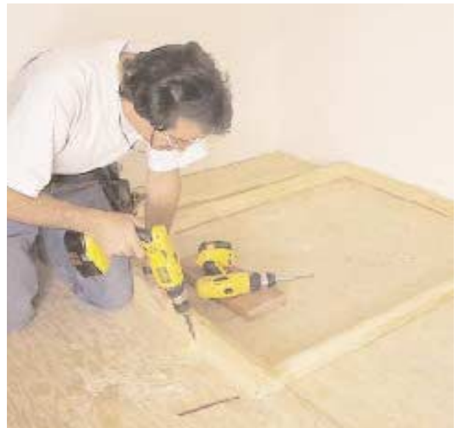
Figure 6. After fastening the back-rabbeted extension jambs to the stool with drywall screws, the author drills pilot holes in the shoulder using a tapered countersink bit (left). He also countersinks the stool so the screws won't interfere with the apron (right).
