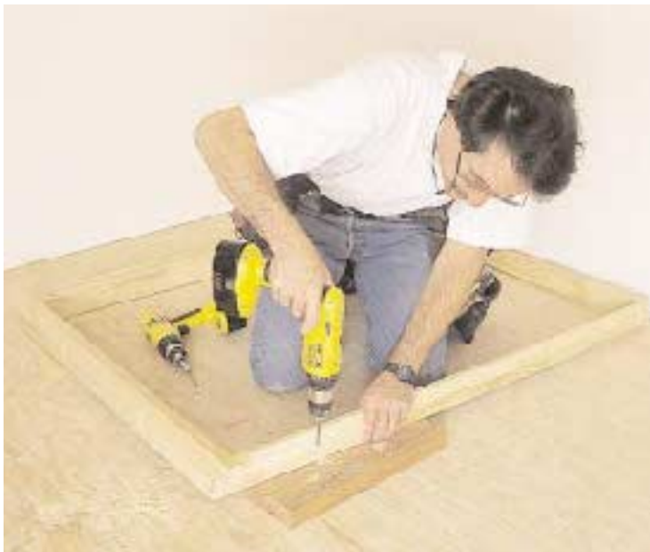
Figure 6. After fastening the back-rabbeted extension jambs to the stool with drywall screws, the author drills pilot holes in the shoulder using a tapered countersink bit (left). He also countersinks the stool so the screws won't interfere with the apron (right).
