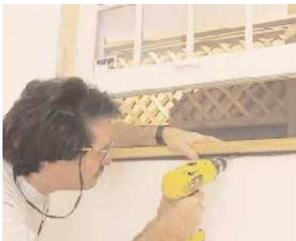
Figure 7. After positioning the preassembled frame against the window jambs (above), screw the extensions through the back-rabbets (above right), and fasten the stool through the countersunk pilot holes (right).
