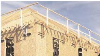
and overhang depth, no part of the guardrail assembly touches any part of the roof, so nothing needs to be removed to complete roof construction. Warranted to meet OSHA requirements for fall protection systems when used according to manufacturer's instructions. Price is \$145 per pair, plus shipping.
